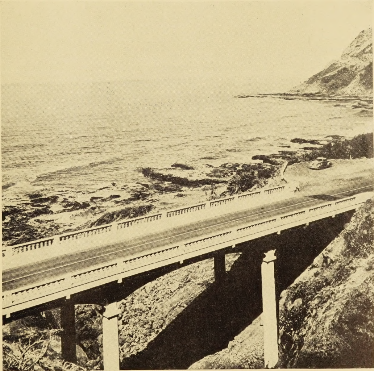
A CONTINUOUS CONCRETE BRIDGE
