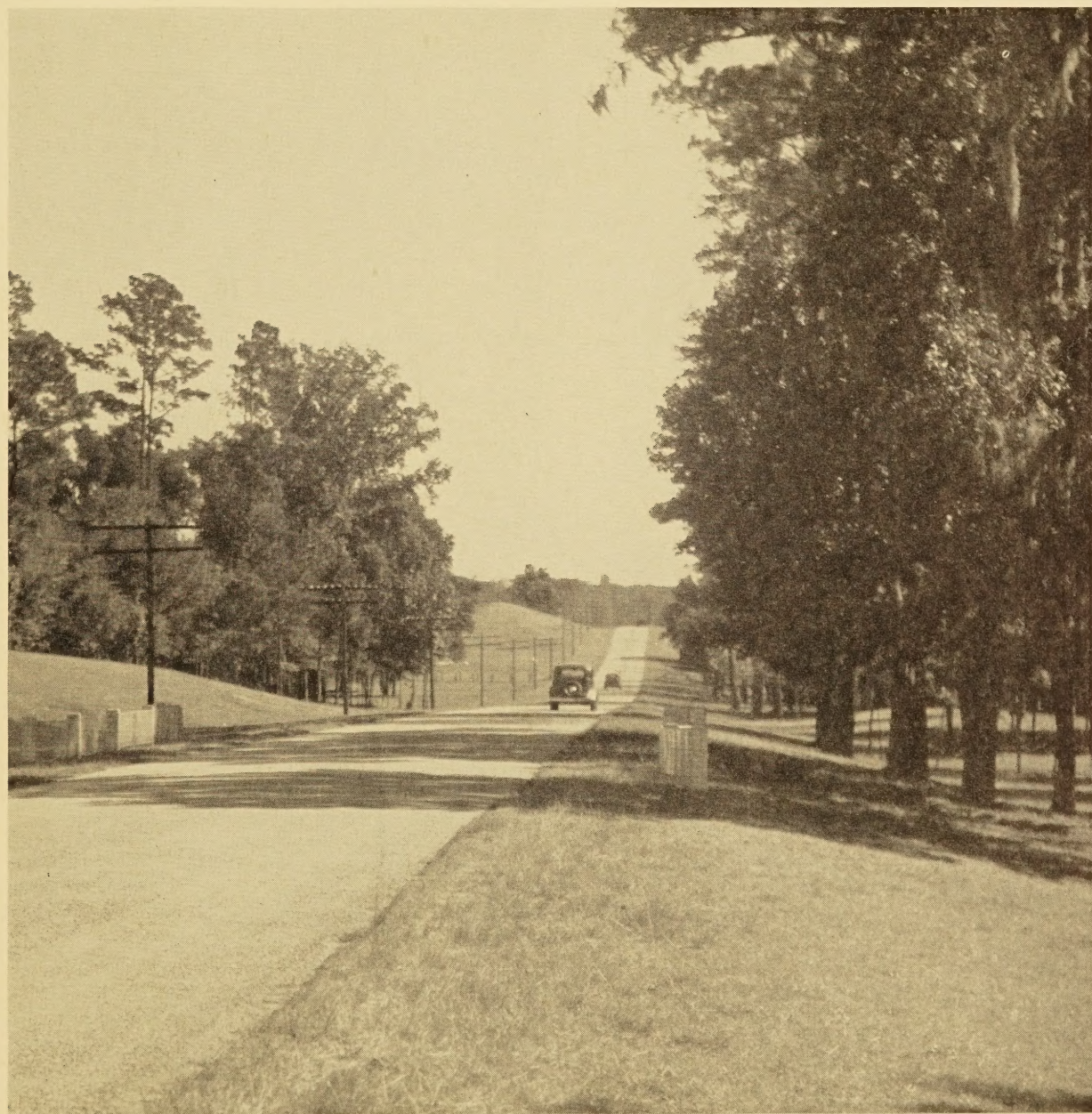
WELL-DESIGNED DRAINAGE CHANNELS ALONG U S 90 IN FLORIDA
