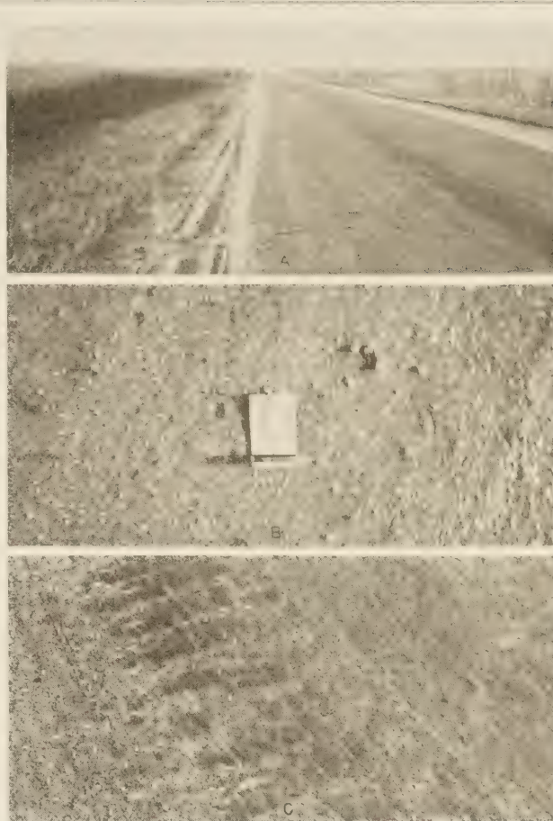
FIGURE 11.—A, CUT-BACK SECTION AFTER RE-TREATMENT. THE GRASS LINE MARKS THE EDGE OF THE ORIGINAL BITUMINOUS MAT AND THE ARROW MARKS THE EDGE OF THE RE-TREATMENT. LOOSE MATERIAL NEAR THE EDGES HAS BEEN WHIPPED TO THE SIDES BY TRAFFIC. B, APPEARANCE OF THE SURFACE IMMEDIATELY AFTER RE-TREATMENT. C, APPEARANCE OF SECTION 9A 3 YEARS AFTER SURFACE TREATMENT. THE DARK STRIP IS THE AREA BETWEEN WHEEL TRACKS AND IS SLIGHTLY RAISED.
