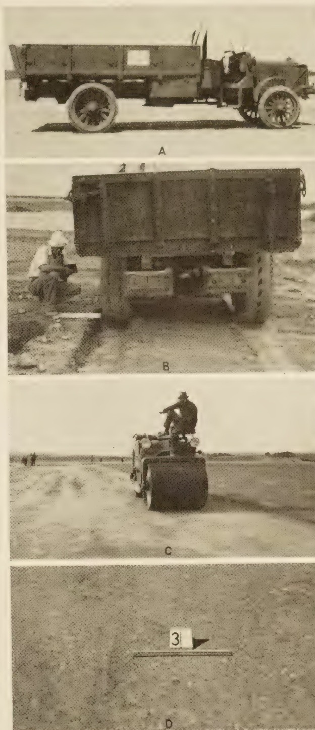
FIGURE 12 - A, CHECKING BASE STABILITY WITH A 12-TON, SOLID-TIRED TRUCK; B, FAILURE DUE TO WEAK SUBGRADE; C, FINAL ROLLING WITH AN 8-TON TANDEM ROLLER, AND D, APPEARANCE OF COMPLETED BASE COURSE.
