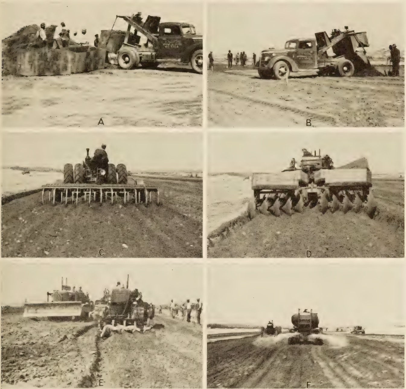
FIGURE 9.—STABILIZATION OF RUNWAYS: A, LOADING BINDER SOIL IN 2-CUBIC YARD BOXES; B, DEPOSITING AND SPREADING BINDER SOIL; C, CUTTING IN BINDER SOIL WITH FIELD CULTIVATOR; D, MIXING WITH TWO-WAY TANDEM DISK HARROW; E, TURNING DISKED MATERIAL WITH FOUR-BOTTOM GANG PLOW; AND F, SPRINKLING DURING MIXING OPERATIONS.
