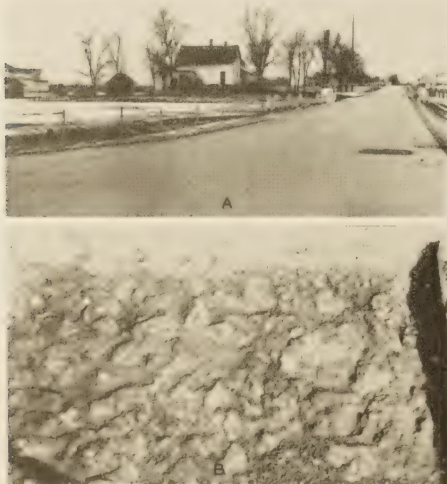
FIGURE 3.—A, GENERAL VIEW OF AN EXCELLENT PAVEMENT, AND B, DETAIL OF THE GOOD WATER-BOUND MACADAM BASE EXPOSED BY REMOVAL OF THE SAMPLE. THE DARK SPOT IN THE RIGHT FOREGROUND IN A IS THE PATCH THAT WAS PLACED AFTER THE REMOVAL OF SAMPLE 11-C-1.
