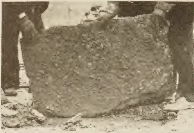
FIGURE 1.—A TYPICAL FIELD SAMPLE OF BITUMINOUS CONCRETE SURFACING.
