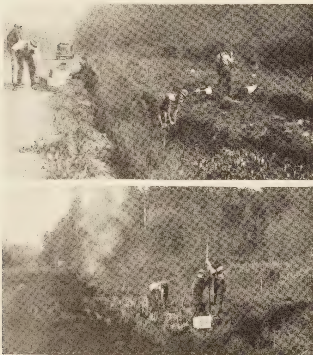
FIGURE 5.—PUNCHING AND LOADING HOLES FOR SWAMP MAT BLASTING.
