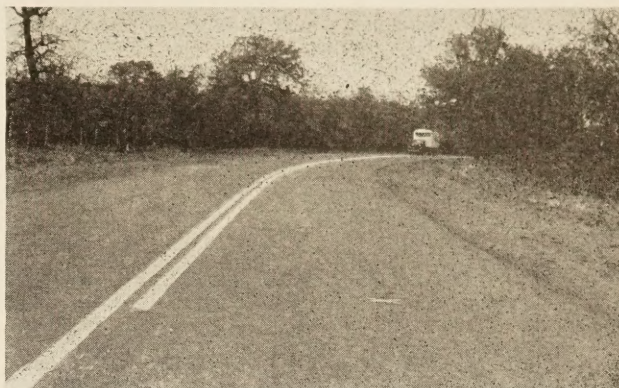
CENTERLINE STRIPE AND DIRECTIONAL STRIPE TO RESTRICT TRAFFIC APPROACHING THE CURVE. THE MARKING WOULD BE MORE EFFECTIVE WERE THE CENTERLINE STRIPE BROKEN INSTEAD OF SOLID OR DIFFERENT IN WIDTH OR COLOR.
