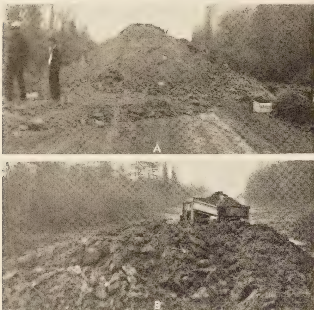
FIGURE 4.—FILL MATERIAL PILED ON ROAD PRIOR TO UNDER-FILL BLASTING. A, MATERIAL FROM UPPER 12 FEET OF BORROW PIT; B, MATERIAL FROM LOWER PART OF BORROW PIT.
