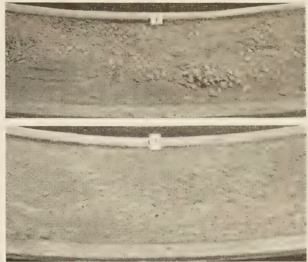
FIGURE 11.—SECTIONS OF TRACK 3 AT 160,000 WHEEL-TRIPS, JUST BEFORE THE FIRST SPRINKLING. UPPER, SECTION 1, WHICH IS ALSO REPRESENTATIVE OF SECTION 2; LOWER, SECTION 3. SECTIONS 4 AND 5 WERE IN SLIGHTLY BETTER CONDITION THAN SECTION 3.
