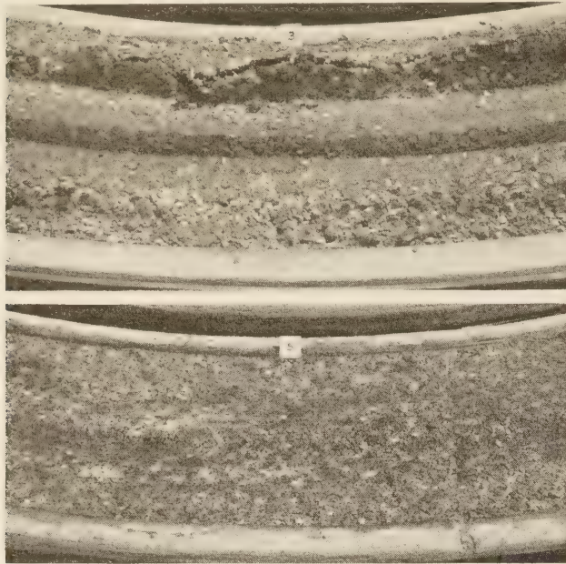
FIGURE 13.—SECTIONS OF TRACK 3 AT THE CONCLUSION OF THE TEST. UPPER, SECTION 3, WHICH IS ALSO REPRESENTATIVE OF SECTION 4; LOWER, SECTION 5, WHICH IS ALSO REPRESENTATIVE OF SECTIONS 1 AND 2.
