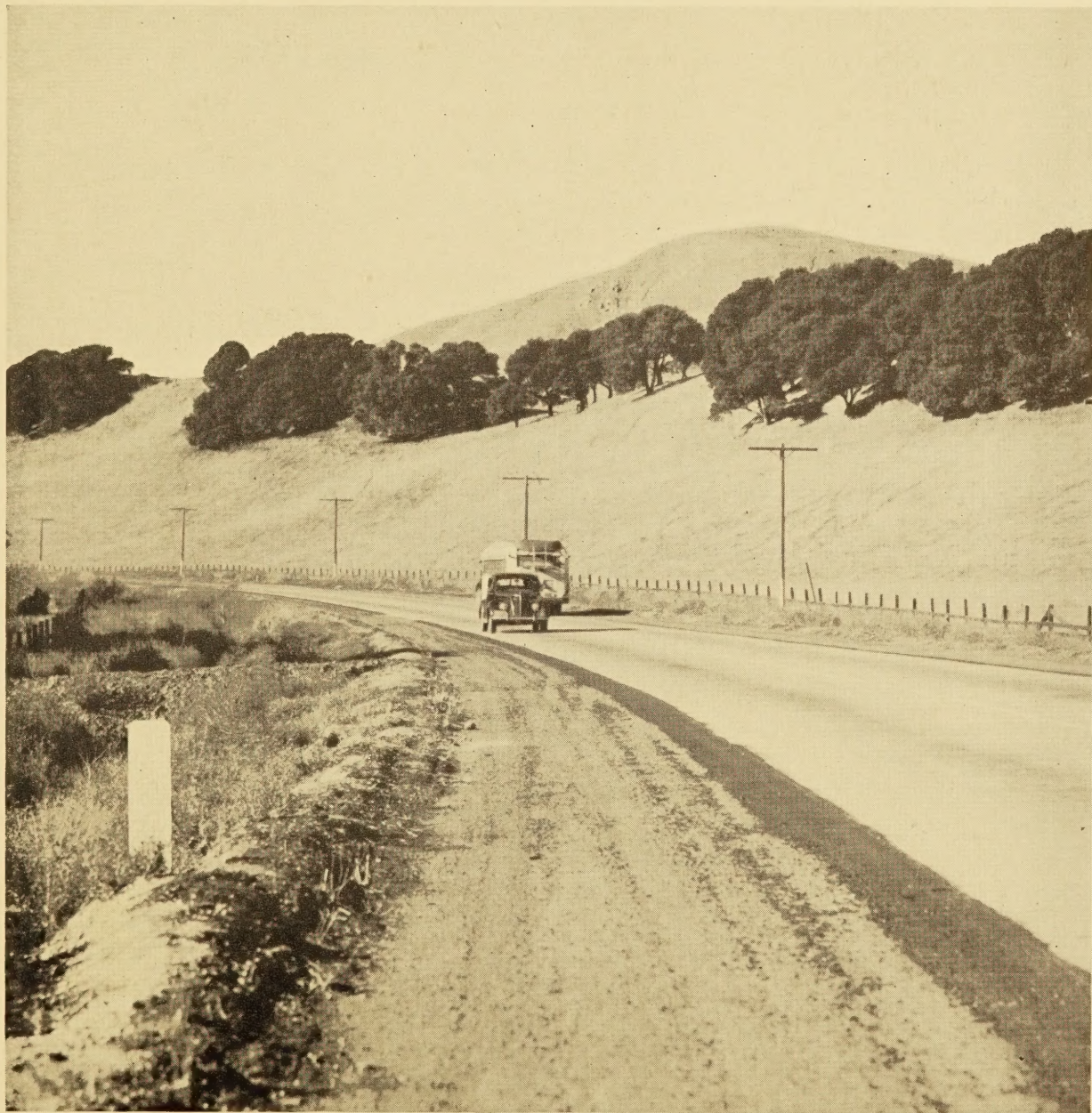
A SECTION OF STATE ROUTE 37 IN CALIFORNIA
