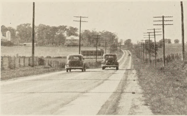
FIGURE 3.—DETECTORS IN PLACE ON A SECTION OF ROAD ON WHICH PASSING PRACTICES WERE OBSERVED.
