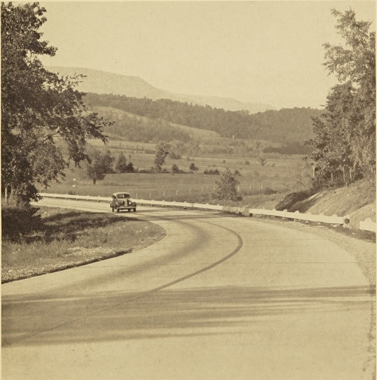
A SECTION OF US 64 IN TENNESSEE
