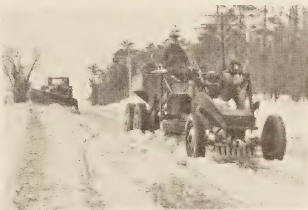
MOTOR GRADERS ARE OFTEN USED FOR LIGHT SNOW-REMOVAL WORK.
