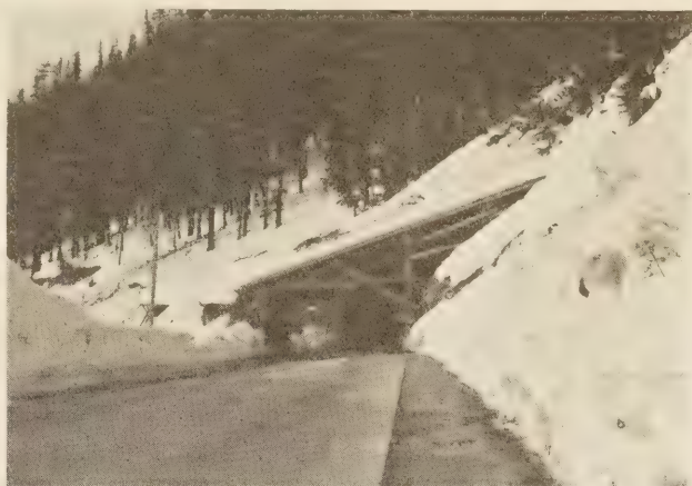
SNOW SHEDS ARE THE MOST PRACTICAL MEANS OF KEEPING ROADS OPEN IN CERTAIN AREAS WHERE SLIDES OCCUR.
