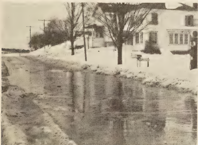
IMPROPER DRAINAGE DURING THE WINTER MAY CAUSE DAMAGE TO THE ROAD AND CREATE A SERIOUS HAZARD TO TRAFFIC.
