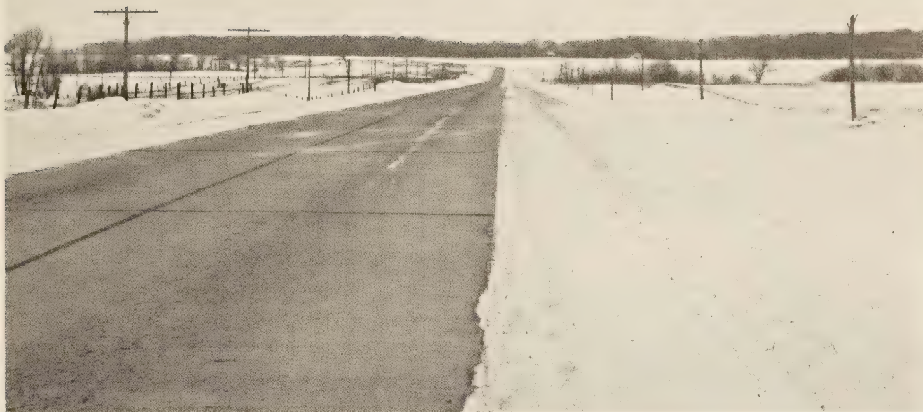
MODERN HIGHWAYS ARE DESIGNED SO AS TO MINIMIZE THE AMOUNT OF SNOW-REMOVAL WORK NEEDED TO KEEP THEM OPEN TO TRAFFIC.
