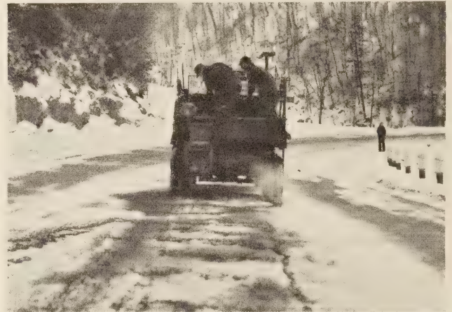
ICY PAVEMENTS ARE MADE SAFER FOR TRAFFIC BY SPREADING SAND OR CINDERS AT DANGEROUS PLACES.
