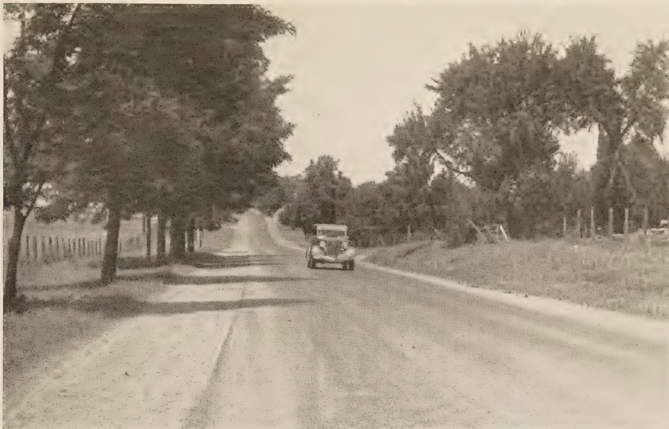
THE WELL-DESIGNED FLEXIBLE-TYPE ROAD ADEQUATELY SERVES MODERN TRAFFIC. THE LOAD-CARRYING CAPACITY OF SUCH A ROAD DEPENDS UPON THE SUPPORTING POWER OF THE SUBGRADE AS WELL AS UPON THE THICKNESS OF THE SURFACE.
