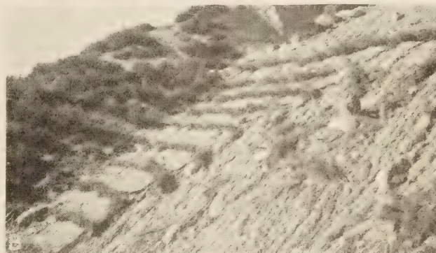
FIGURE 9.—DAMAGED FILLS THAT HAD BEEN PROTECTED BY BRUSH WATTLES (METHOD C).
