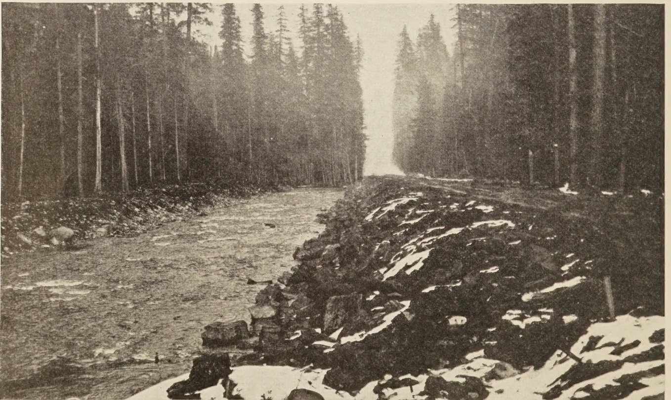
FIGURE 6.—PROGRESS DURING CONSTRUCTION OF A CHANNEL CHANGE.
