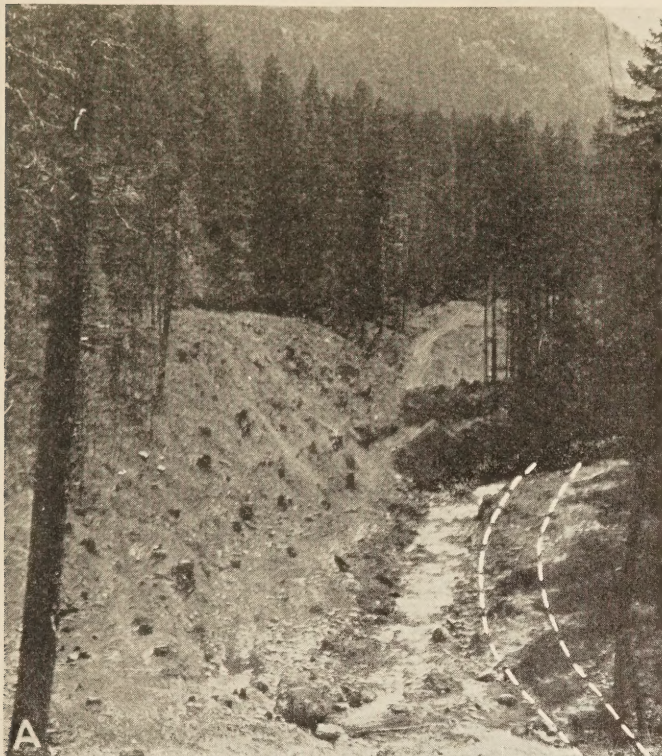
FIGURE 1.—ORIGINAL TERRAIN AND COMPLETED ROAD AND CHANNEL CHANGE. A, THE DOTTED LINES MARK THE CHANNEL CHANGE LOCATION. B, THE HIGHWAY FILL SLOPE IS RIPRAPPED AT THE BOTTOM WHERE IT SERVES AS ONE BANK OF THE STREAM.
