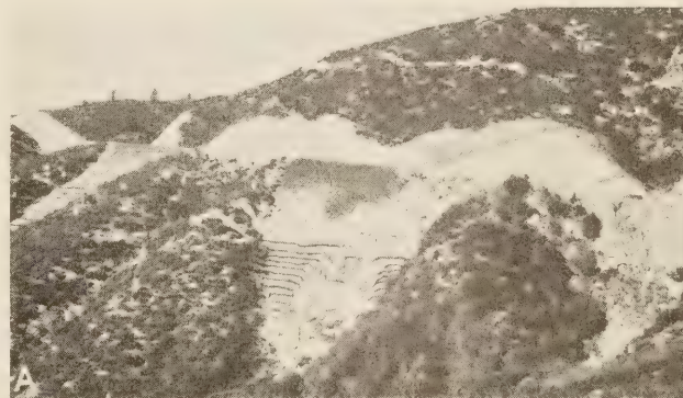
FIGURE 8.—SECTIONS OF FILL SLOPES ABOUT 70 FEET BELOW GRADE. A; EROSION ON AN UNPROTECTED FILL. B; A FILL PROTECTED ACCORDING TO METHOD A.
