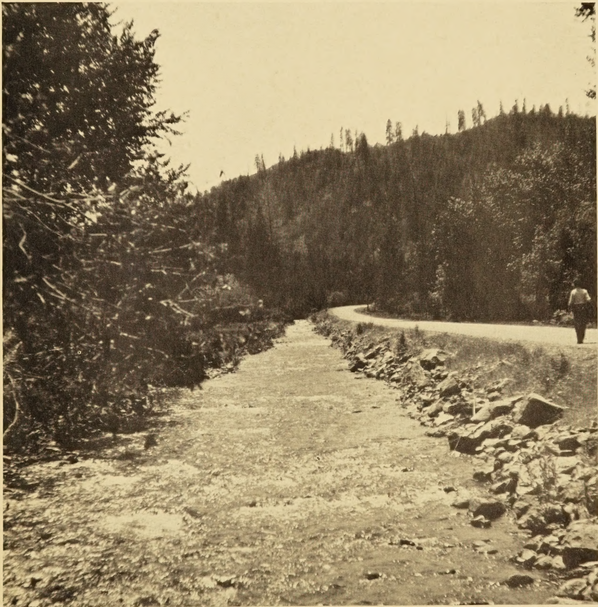
CHANNEL CHANGE ADJACENT TO FOREST HIGHWAY IN OREGON
