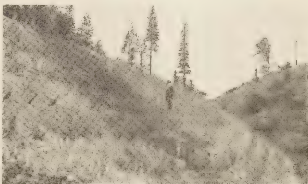
FIGURE 4.—APPEARANCE OF A FILL 9 MONTHS AFTER WILLOW CUTTINGS HAD BEEN PLANTED.
