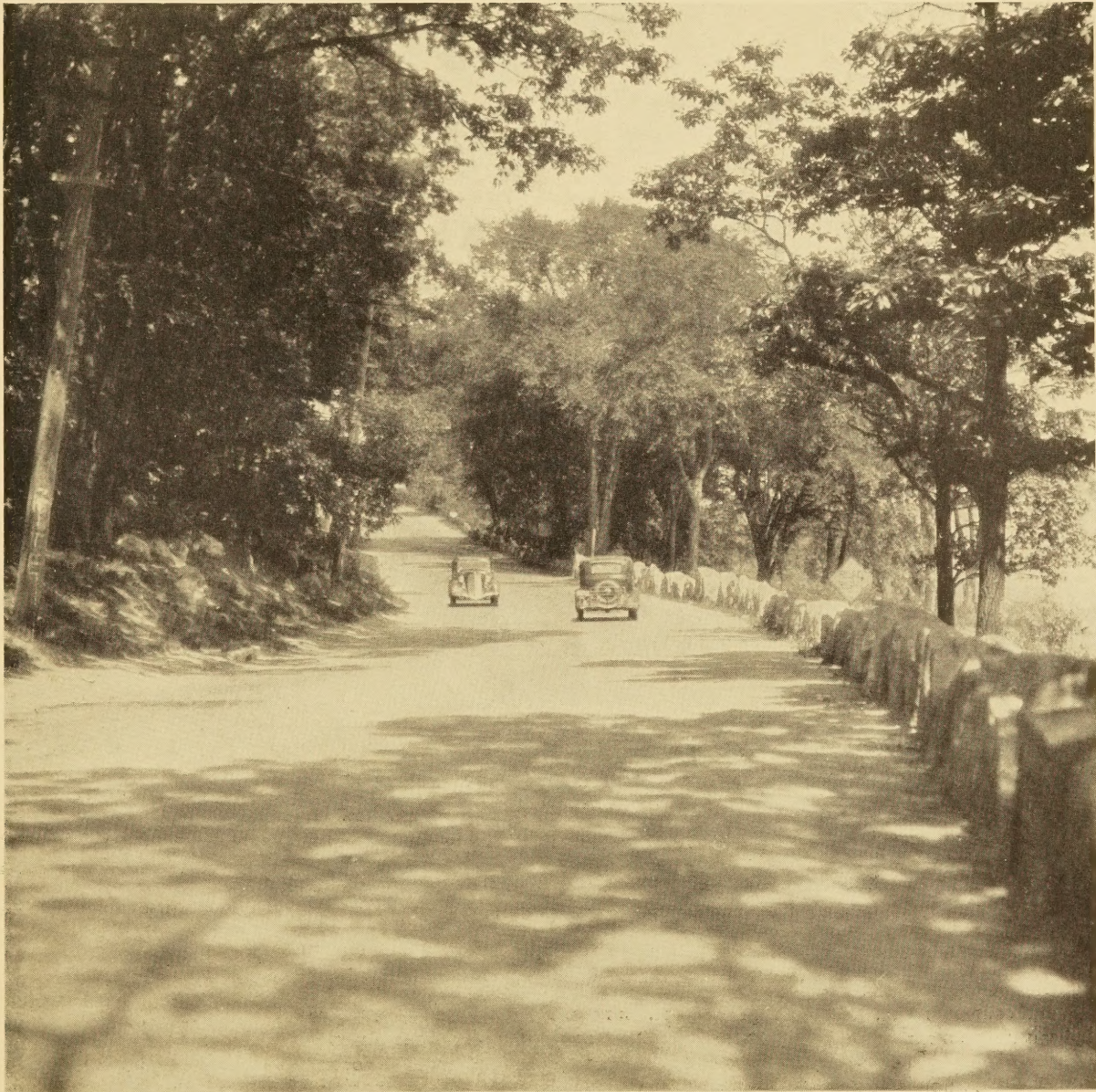
A SECTION OF BITUMINOUS MACADAM ON STATE ROUTE 127 IN MASSACHUSETTS
