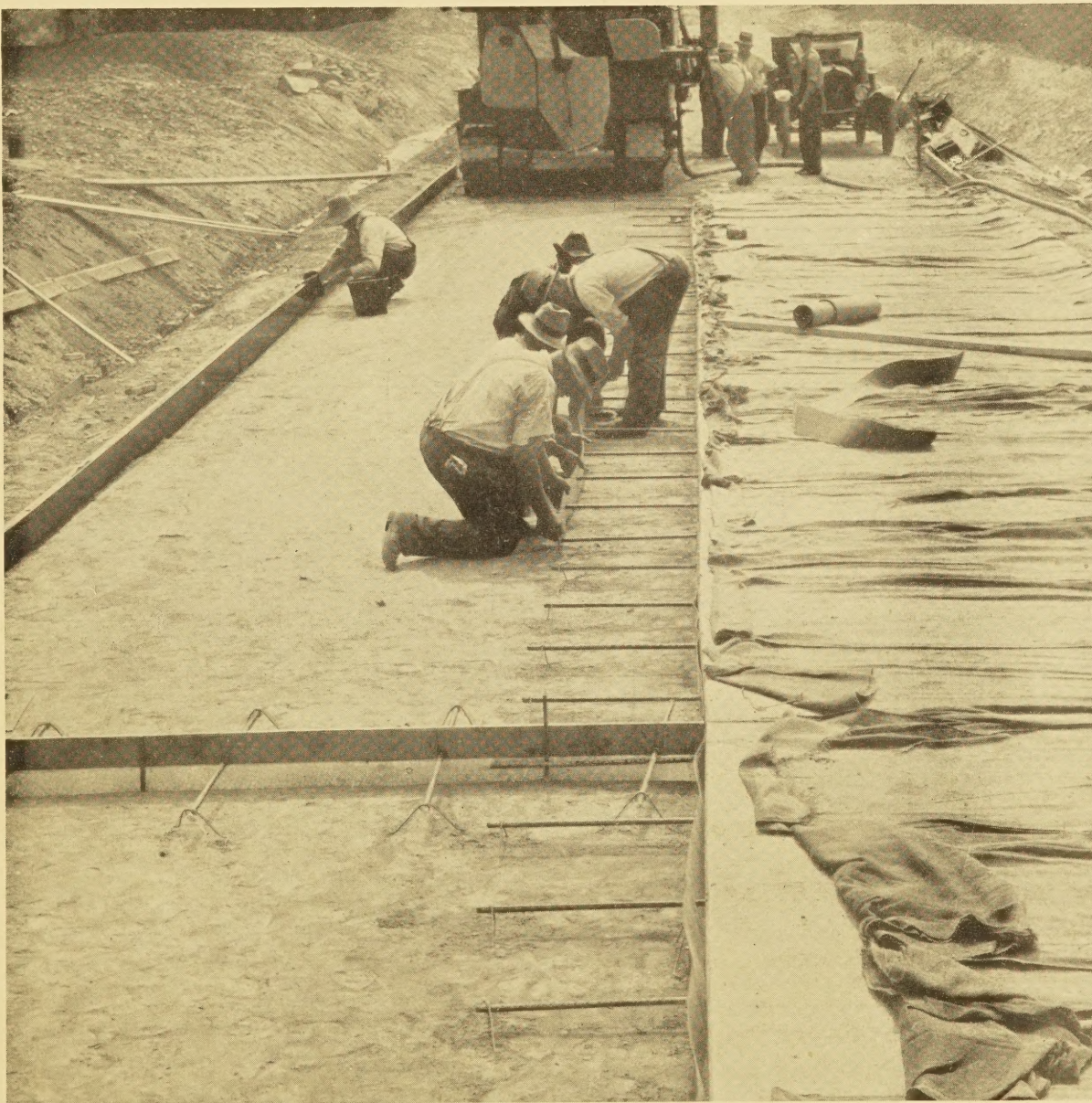
PLACING TARRED FELT ALONG A LONGITUDINAL JOINT
