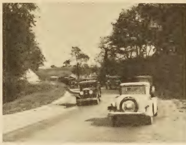
A METHOD OF INCREASING SIGHT DISTANCE ON SHARP CURVES. IN THIS CASE CONDITIONS ARE IMPROVED BUT ARE STILL DANGEROUS.
