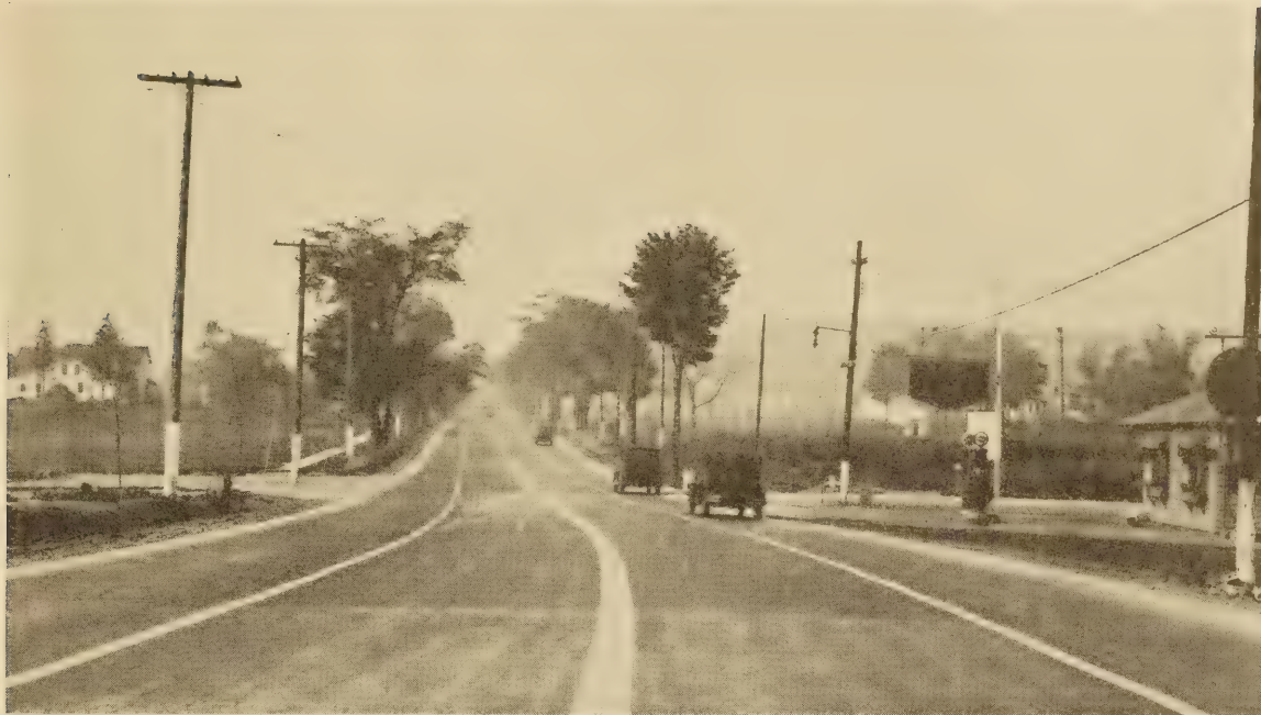
MANY SERIOUS ACCIDENTS OCCUR ON WIDE AND STRAIGHT ROADWAYS WITH LANES MARKED. THE PRESENT TENDENCY IN DESIGNING 4-LANE ROADWAYS IS TOWARD SEPARATION OF TRAFFIC MOVING IN OPPOSITE DIRECTIONS BY A CENTER PARKWAY
