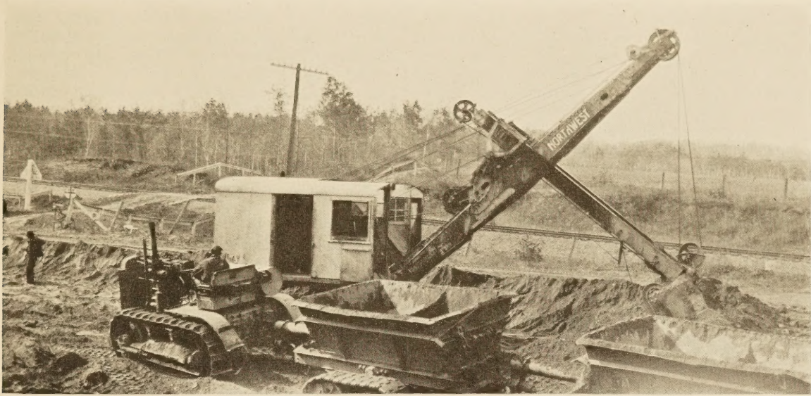
SHOVEL LOADING TWO 5-CUBIC-YARD WAGONS.
