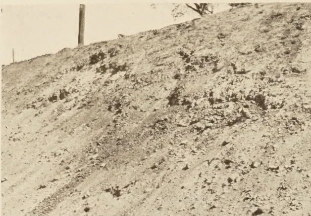
DRESSING SLOPES BY HAND AND THE SAME SLOPE FIVE DAYS LATER AS WASHED BY RAIN. TOO MUCH REFINEMENT INCREASES COST WITHOUT PRODUCING ADVANTAGES.
