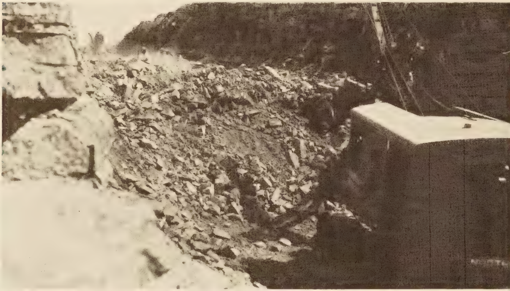
SAME ROCK LEDGE AS ABOVE, WELL BROKEN BY PROPER BLASTING.
