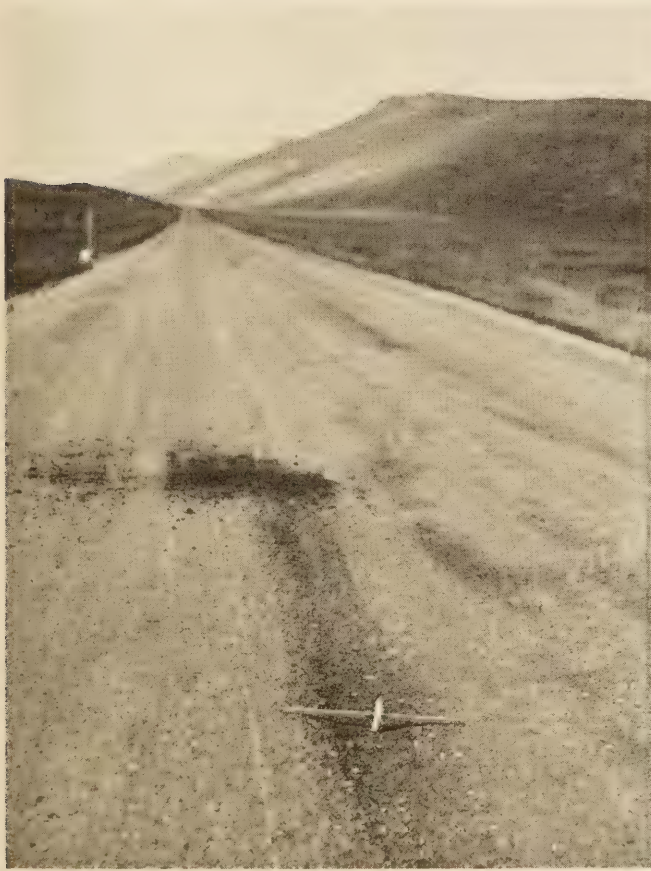
TYPICAL EXAMPLES OF RAVELING OF GROUP 3 SURFACES HAVING A LOW OIL CONTENT AND NO SEAL COAT OR SURFACE TREATMENT TO PREVENT LOSS OF AGGREGATE.
