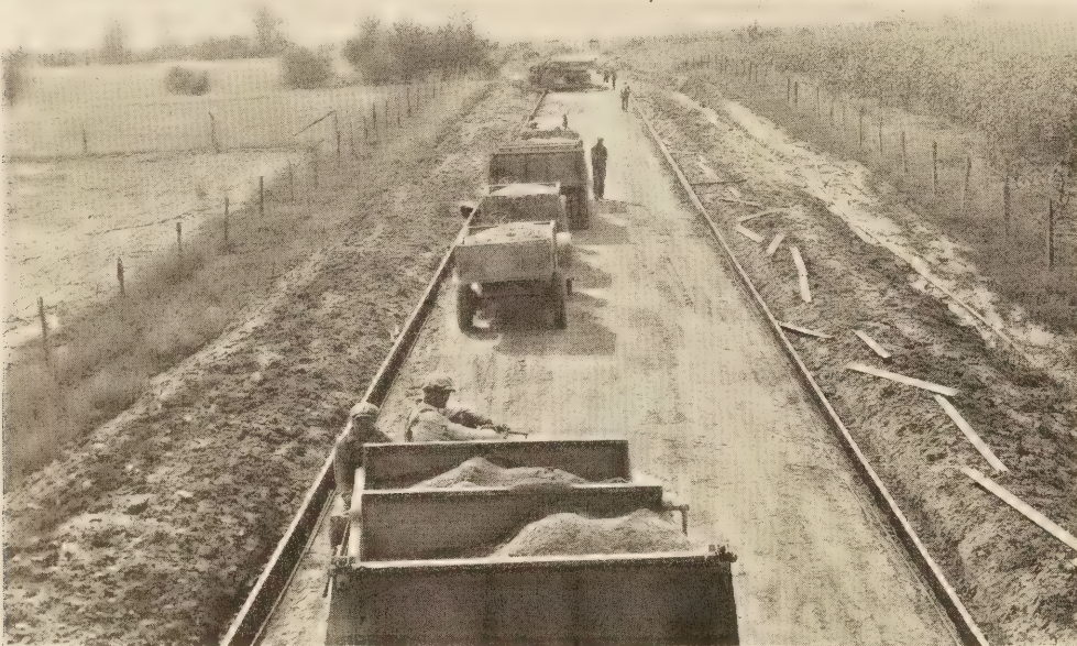
TRUCKS READY TO BACK TO PAVER.
