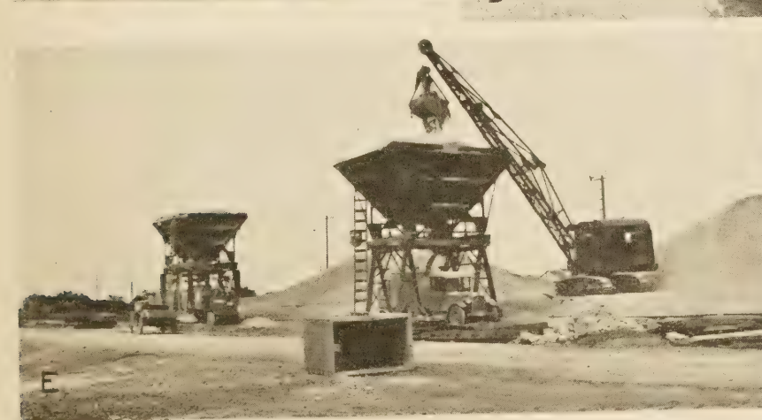
A, crane unloading aggregates from cars to batcher bins or stockpiles as conditions require; B, unloading cement from cars to batch compartments of trucks; C, bin for handling bulk cement and batcher plant; D, batcher plant; E, a good plant arrangement; F, handling bulk cement in "buggies."
