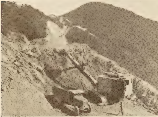
EXAMPLES OF CORRECT "SPOTTING" OF TRUCKS FOR LOADING WITH SHORT SWING OF SHOVEL.
