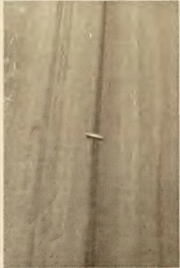
GENERAL VIEW AND DETAIL OF A SURFACE OF GROUP 1 WHICH WAS HIGHLY UNSTABLE DUE TO A HIGH COMBINED OIL AND WATER CONTENT. AGE APPROXIMATELY ONE YEAR AT TIME OF INSPECTION. NOTE TIRE MARKS AND FOOT TRACKS ON THIS SURFACE.
