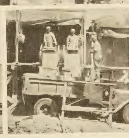
A, crane unloading aggregates from cars to batcher bins or stockpiles as conditions require; B, unloading cement from cars to batch compartments of trucks; C, bin for handling bulk cement and batcher plant; D, batcher plant; E, a good plant arrangement; F, handling bulk cement in "buggies."
