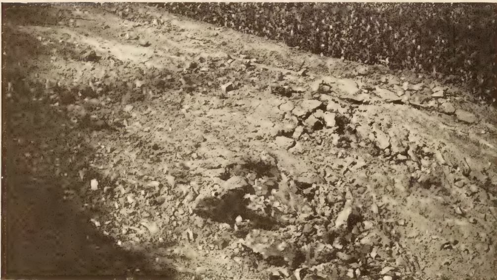
APPEARANCE OF GROUND AFTER A SATISFACTORY BLAST. MATERIAL WELL BROKEN BUT NOT SCATTERED.
