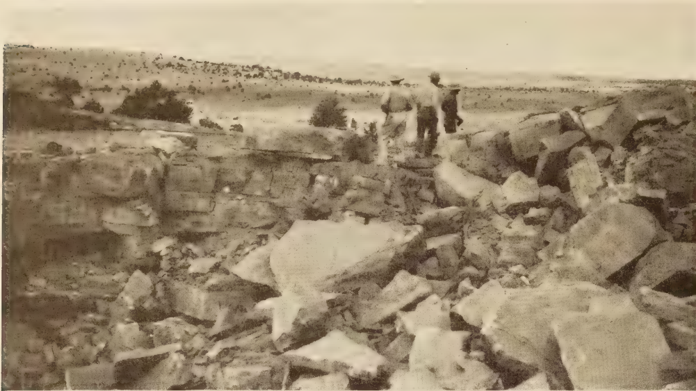
IMPROPER SPACING AND LOADING OF DRILL HOLES RESULTED IN MATERIAL HARD TO LOAD.
