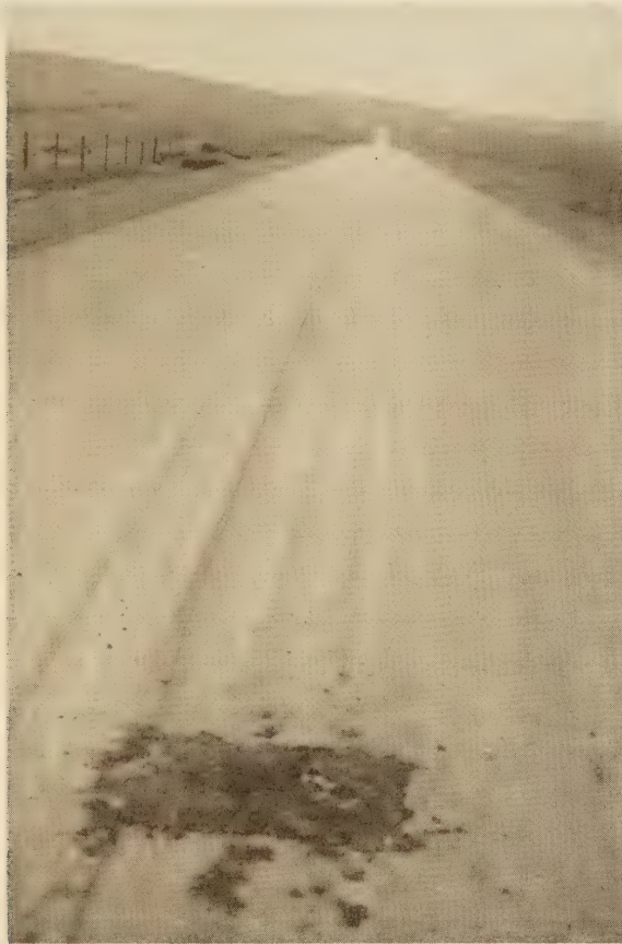
GENERAL VIEW AND DETAIL OF A SURFACE OF GROUP 1 WHICH WAS HIGHLY UNSTABLE DUE TO A HIGH COMBINED OIL AND WATER CONTENT. AGE APPROXIMATELY ONE YEAR AT TIME OF INSPECTION. NOTE TIRE MARKS AND FOOT TRACKS ON THIS SURFACE.
