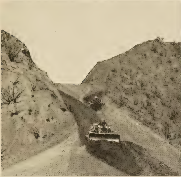
CUT ILLUSTRATED ON COVER PAGE AT AN ADVANCED STAGE OF CONSTRUCTION.
