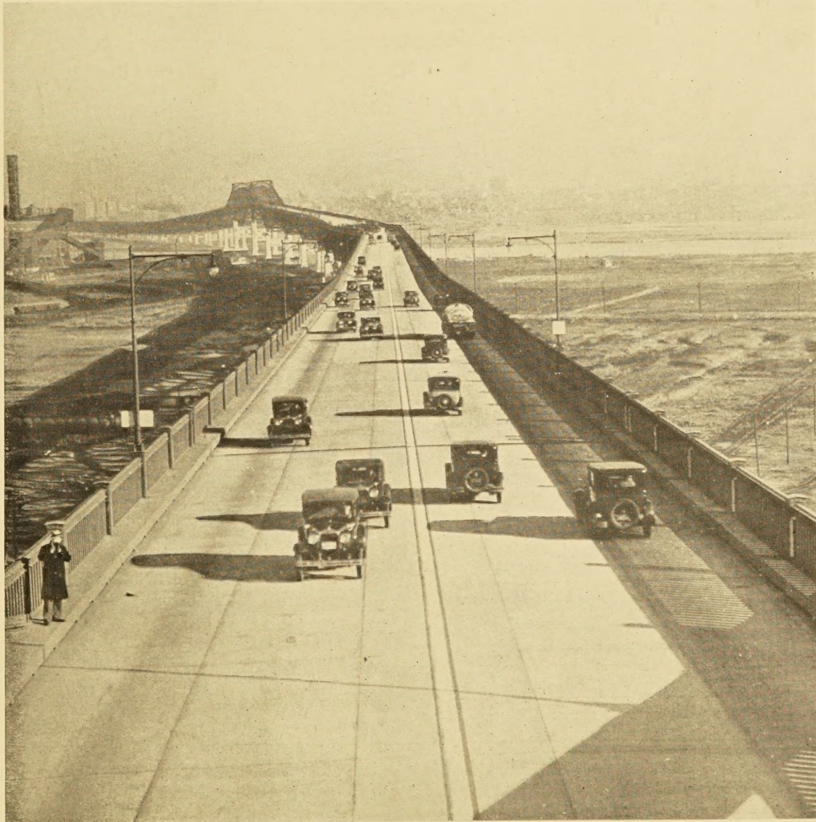
THE NEW JERSEY HIGH-LEVEL VIADUCT
