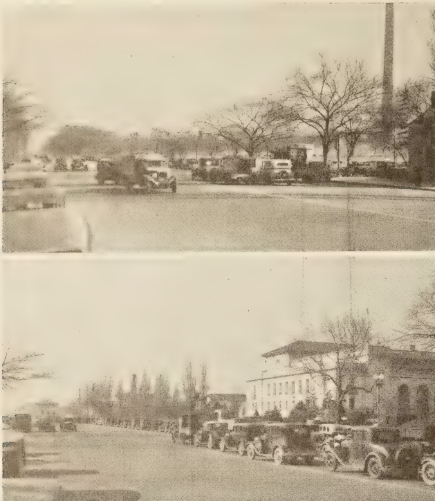
FIGURE 6.—LONG LIGHT INTERVALS UNDER FIXED CONTROL RESULTED IN WAITING LINES AND HIGH AVERAGE VEHICLE TIME.
