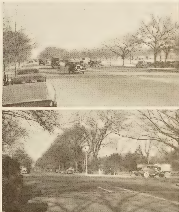
FIGURE 7.—(UPPER) CONDITION UNDER WHICH TRAFFIC ACTUATED CONTROL IS EFFECTIVE AND (LOWER) TYPE OF TRAFFIC WHICH WILL HOLD THE GREEN LIGHT UNLESS "VEHICLE INTERVAL" IS SHORT AND RESULT IN INCREASED AVERAGE VEHICLE TIME.
