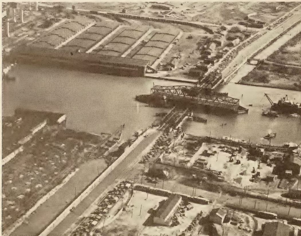
TRAFFIC DELAYED ON COMMUNIPAW AVENUE AS A RESULT OF BRIDGE OPENING.
