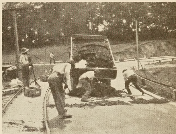
FIGURE 1.—LAYING SURFACE MIXTURE FOR STABILITY EXPERIMENTS.
