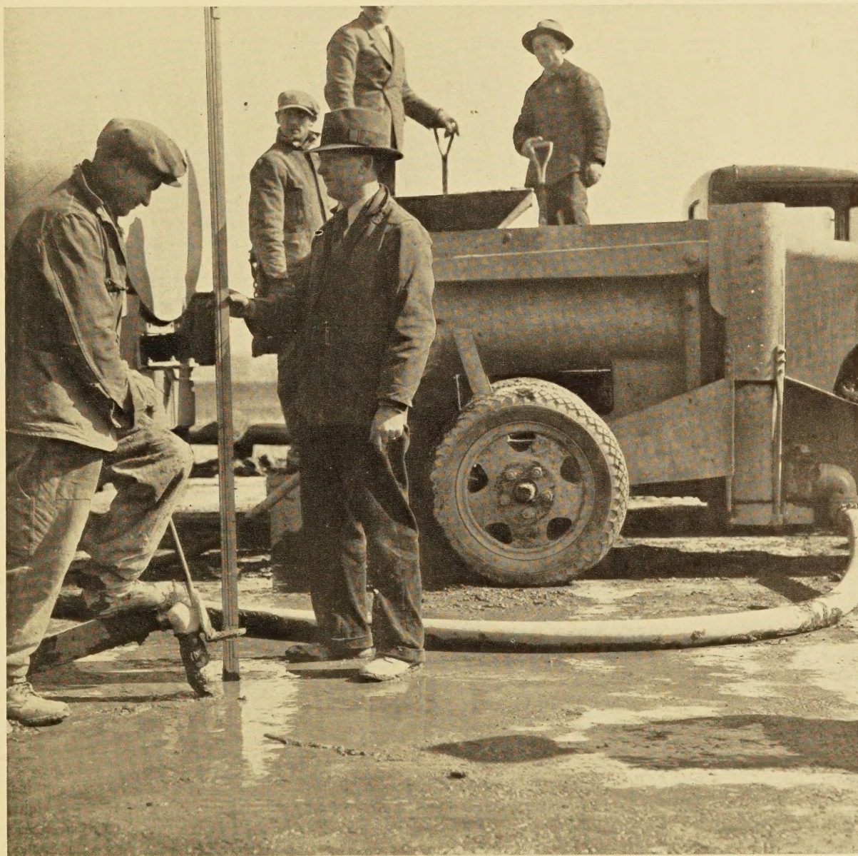
RAISING PAVEMENT BY MUD JACKING
