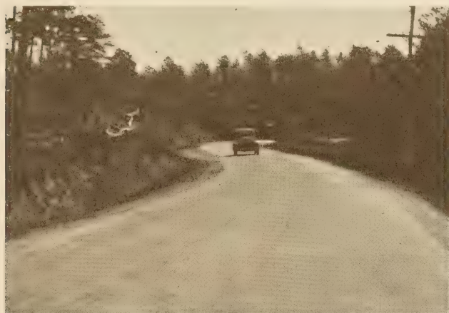
FIGURE 10.—GENERAL VIEW OF NORTH END OF PROJECT, WHICH WAS LOCATED IN FAIRLY ROUGH COUNTRY
