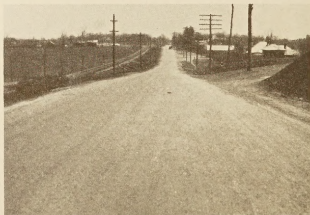
FIGURE 9.—TYPICAL APPEARANCE OF SECTION 11 AFTER APPLICATION OF THE NONSKID TREATMENT
