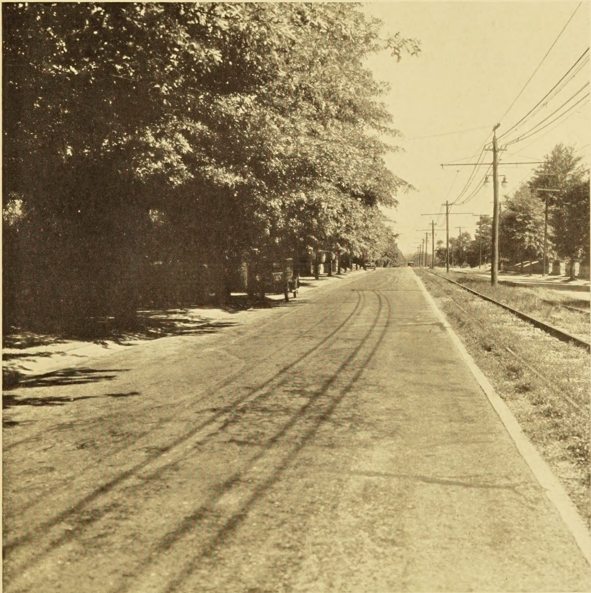
A BITUMINOUS CONCRETE ROAD ON ITS TWENTIETH BIRTHDAY
