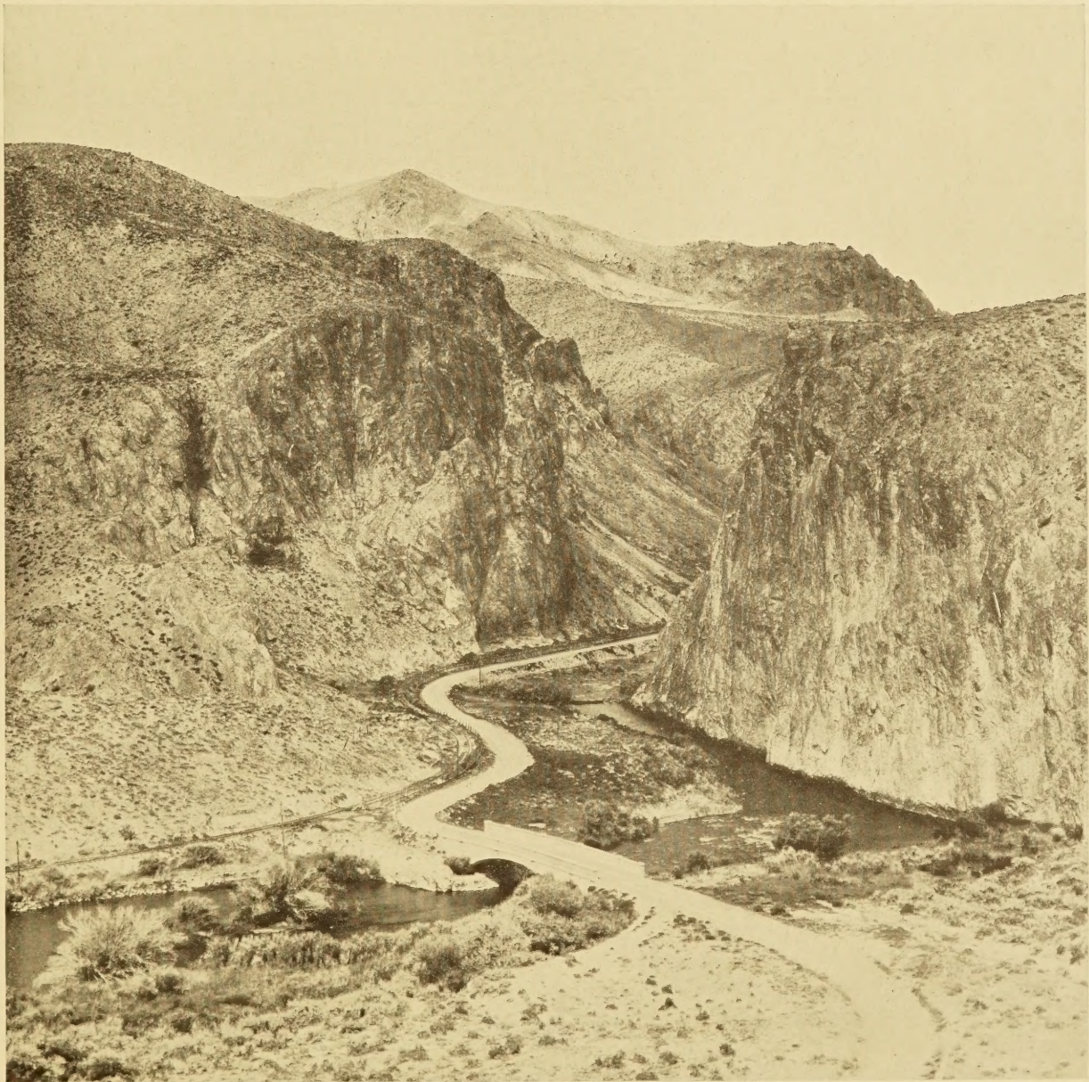
HIGHWAY ENTERING WILSON CANYON IN NEVADA
