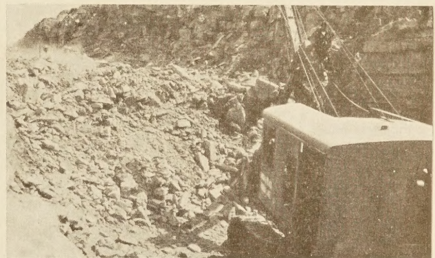
FIGURE 4.—ALMOST ANY ROCK, WHETHER STRATIFIED OR MASSIVE, AND NO MATTER HOW HARD OR TOUGH, CAN BE SO THOROUGHLY BLASTED THAT IT CAN BE HANDLED BY THE SHOVEL AT ABOUT THE SAME RATE AS GOOD COMMON. THIS IS THE SAME KIND OF ROCK AS IS SHOWN IN FIGURE 3
