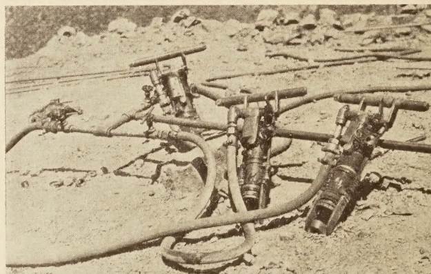
FIGURE 8.—GENERAL TYPE OF JACKHAMMER DRILLS USED IN HIGHWAY WORK
