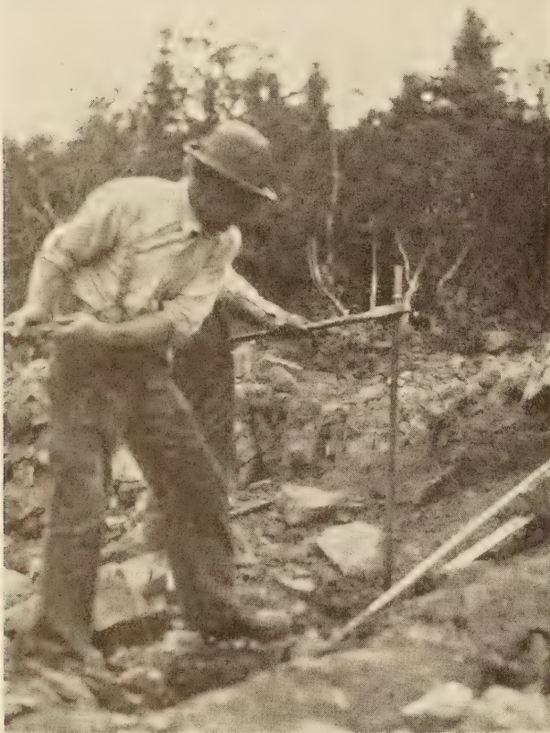
FIGURE 9.—IN SOME ROCK AN INEXPERIENCED OR CARELESS OPERATOR WILL SPEND MUCH OF HIS TIME REMOVING STUCK STEEL. POOR SHARPENING EQUIPMENT OR A CARELESS BLACKSMITH WILL INTENSIFY THIS TROUBLE
