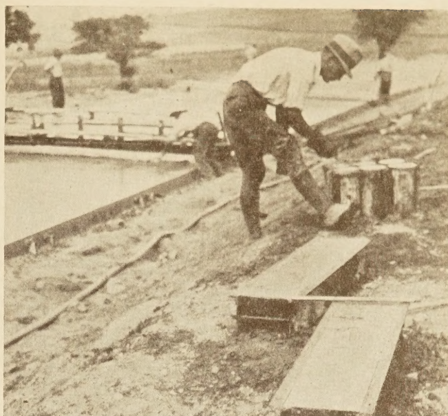
CYLINDERS WERE MADE ACCORDING TO THE A. S. T. M. METHODS. BEAMS WERE RODDED ONLY AT THE EDGES WITHOUT DISTURBING THE CENTER MASS OF THE CONCRETE.
