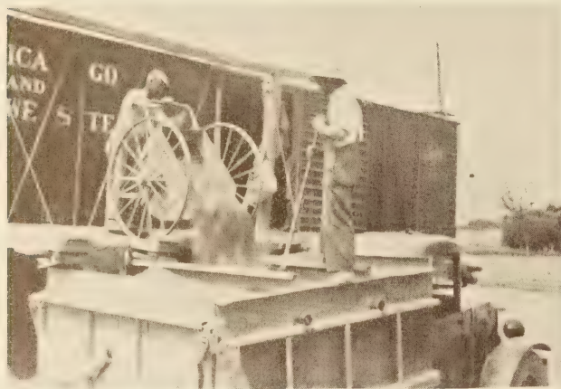
FIGURE 10.—LOCAL PIT PLANT LAYOUT EQUIPPED FOR PRODUCING THREE SIZES OF COARSE AGGREGATE FOR WISCONSIN STATE-AID PROJECT 2926
