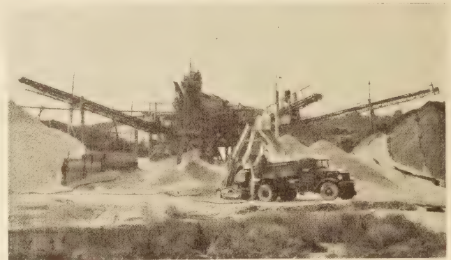
FIGURE 10.—LOCAL PIT PLANT LAYOUT EQUIPPED FOR PRODUCING THREE SIZES OF COARSE AGGREGATE FOR WISCONSIN STATE-AID PROJECT 2926
