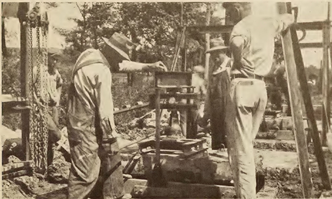
FIGURE 9.—TESTING SLAB FOR FLEXURAL STRENGTH
