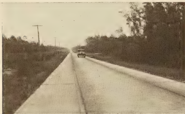
FIGURE 61.—THREE-INCH GROUTED BRICK ROAD CONSTRUCTED ABOUT 1916 ON GROUP A-3 SUBGRADE IN FLORIDA. STILL IN SERVICE. CONCRETE SHOULDERS CONSTRUCTED IN 1921
