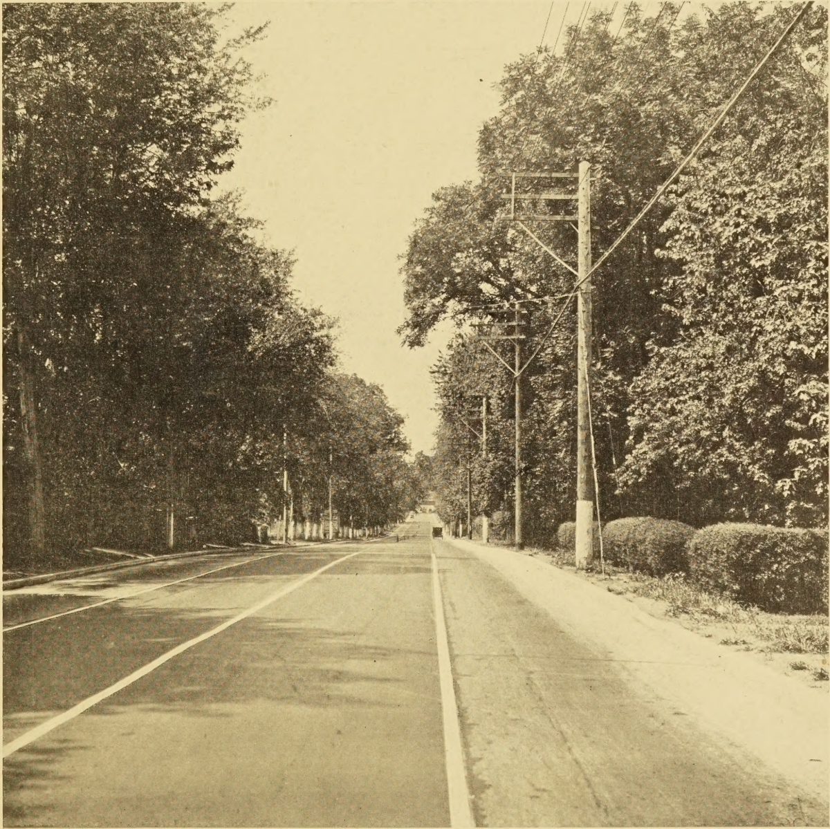
A FOUR-LANE HIGHWAY IN PENNSYLVANIA COURTESY OF PENNSYLVANIA DEPARTMENT OF HIGHWAYS
