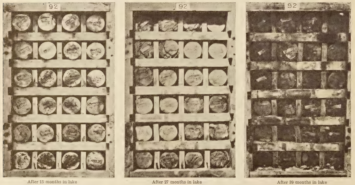
FIGURE 4.—CONDITION OF 1:2:4 CONCRETE CYLINDERS OF MEDIUM CONSISTENCY (BATCH 14, CRATE 92) AFTER 15, 27, AND 39 MONTHS IN MEDICINE LAKE, S. DAK. CURING AND TREATMENT SAME AS IN FIGURE 1
