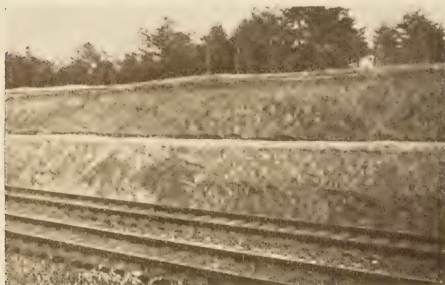
FIGURE 14.—TERRACING OF FACES OF RAILWAY CUT IN CLAY, BETWEEN WASHINGTON AND BALTIMORE. SURFACE DRAINAGE IS PROVIDED FOR ON EACH TERRACE. ONE OF THE METHODS USED TO PREVENT SLIDING IN CUTS
