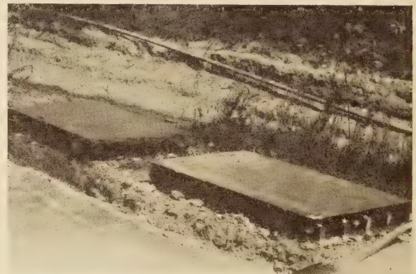
BEAMS UNDER CURE
