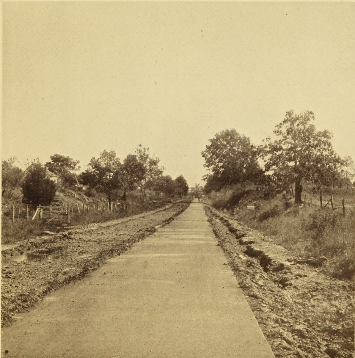
TEST SECTION ON TENNESSEE CONCRETE-CURING PROJECT
