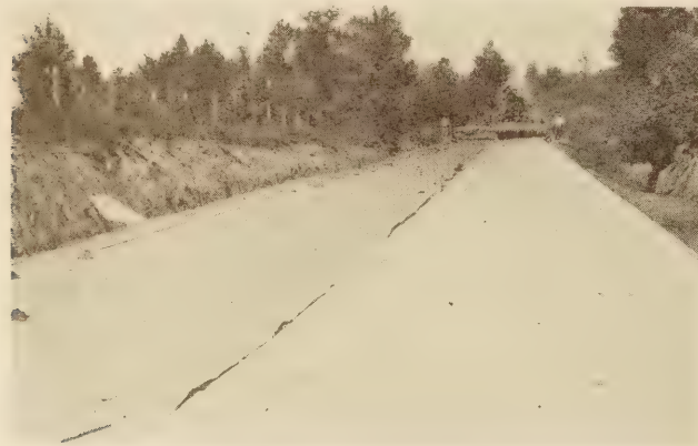
SISALKRAFT PAPER ON RESEARCH SIDE OF LONGITUDINAL JOINT
