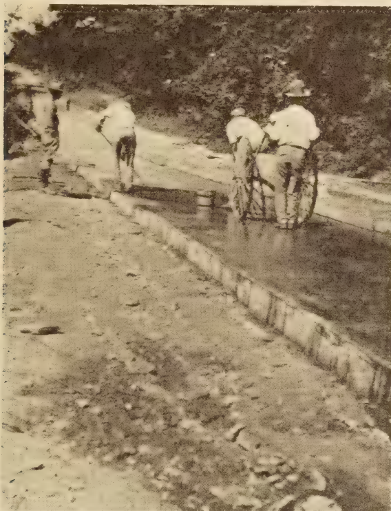
APPLYING SODIUM SILICATE TO SURFACE OF PAVEMENT
