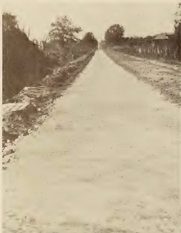
APPEARANCE OF FRESHLY SPREAD CALCIUM CHLORIDE
