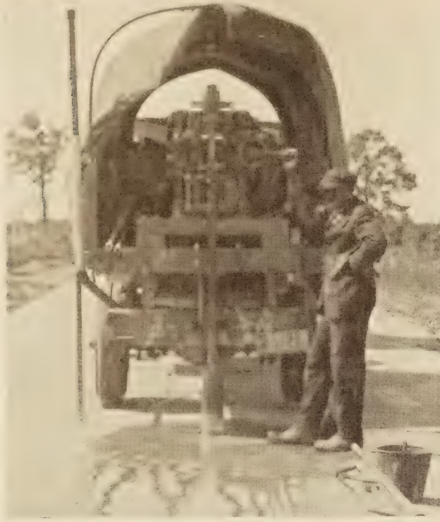
DRILLING CORES FOR COMPRESSION TESTS
