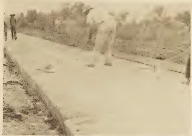
SPREADING CALCIUM CHLORIDE ON PAVEMENT
