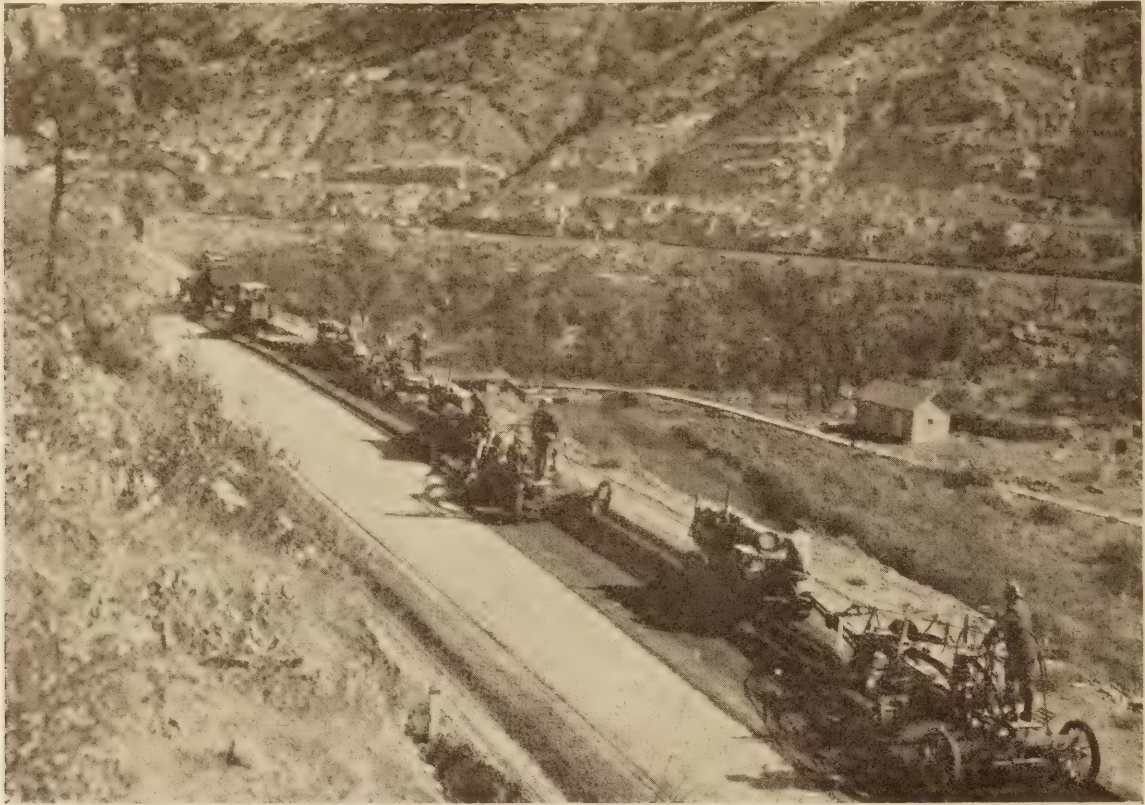
CONSTRUCTING A MIXED-IN-PLACE SURFACE. APPLYING BITUMINOUS MATERIAL, DISKING, AND MIXING
