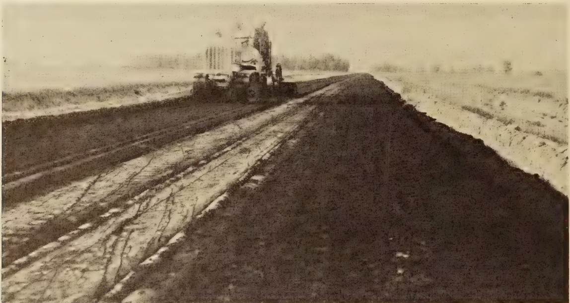
94 PER CENT ROAD OIL CUT BACK WITH KEROSENE MIXED IN PLACE WITH BLOW-SAND SOIL
