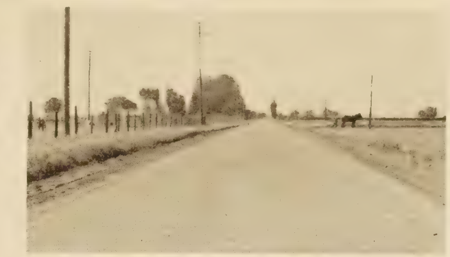
AN OIL-TREATED ROAD IN FRESNO COUNTY, CALIF.
