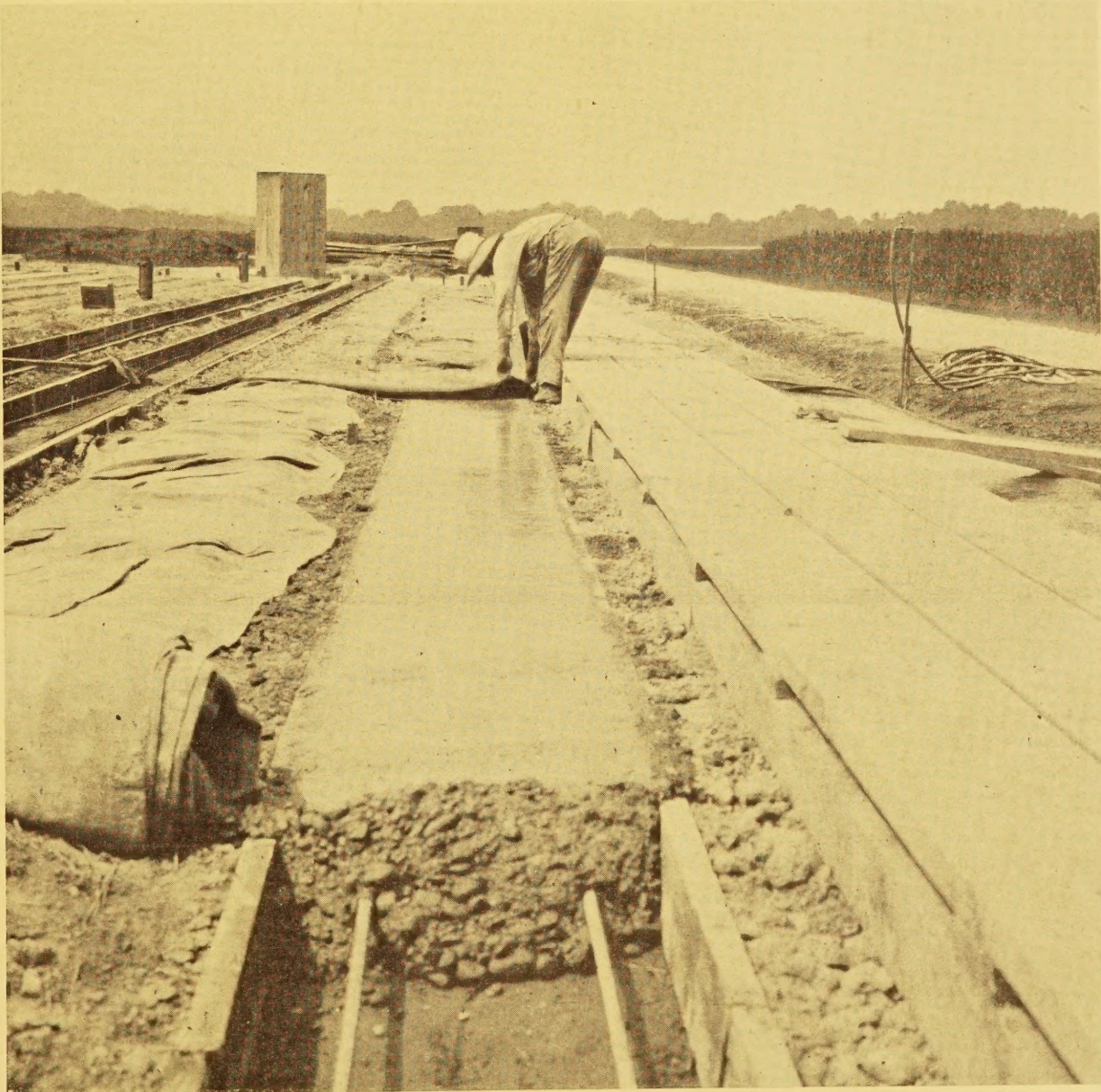
PLACING WET BURLAP IN ARLINGTON CURING EXPERIMENTS
