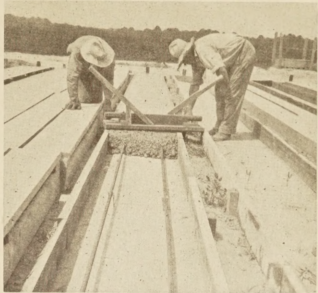
FIGURE 1.—FINISHING A SECTION CONTAINING \frac{3}{4} -INCH DEFORMED BARS
