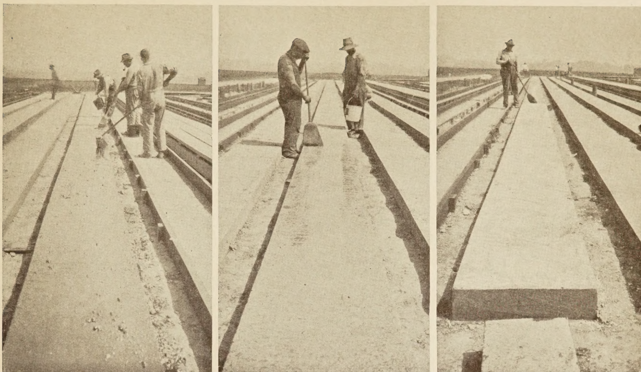
Applying tar to the surface approximately 24 hours after placing
