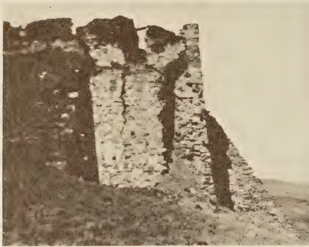
FIGURE 16.—RETAINING WALL ON A HILL WEST OF THE BOSPORUS NORTH OF CONSTANTINOPLE
