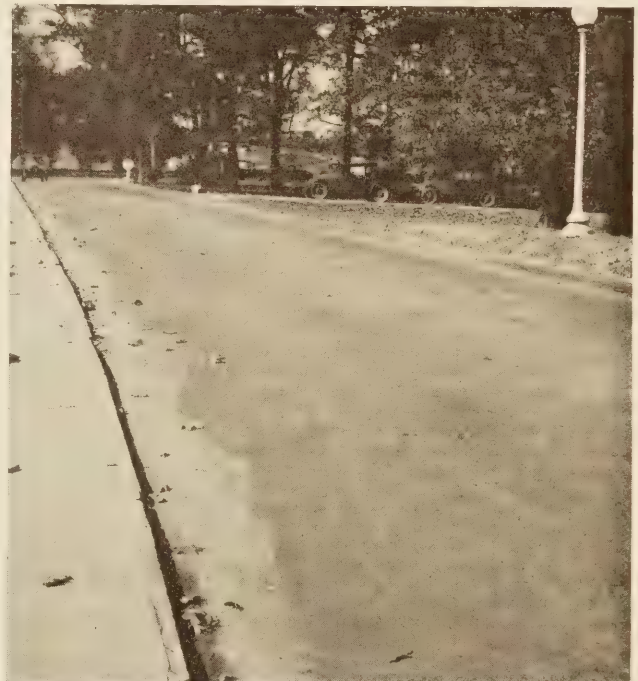
FIGURE 9.—GENERAL VIEW OF LOCATION AND PRESENT CONDITION OF SECTION 8
