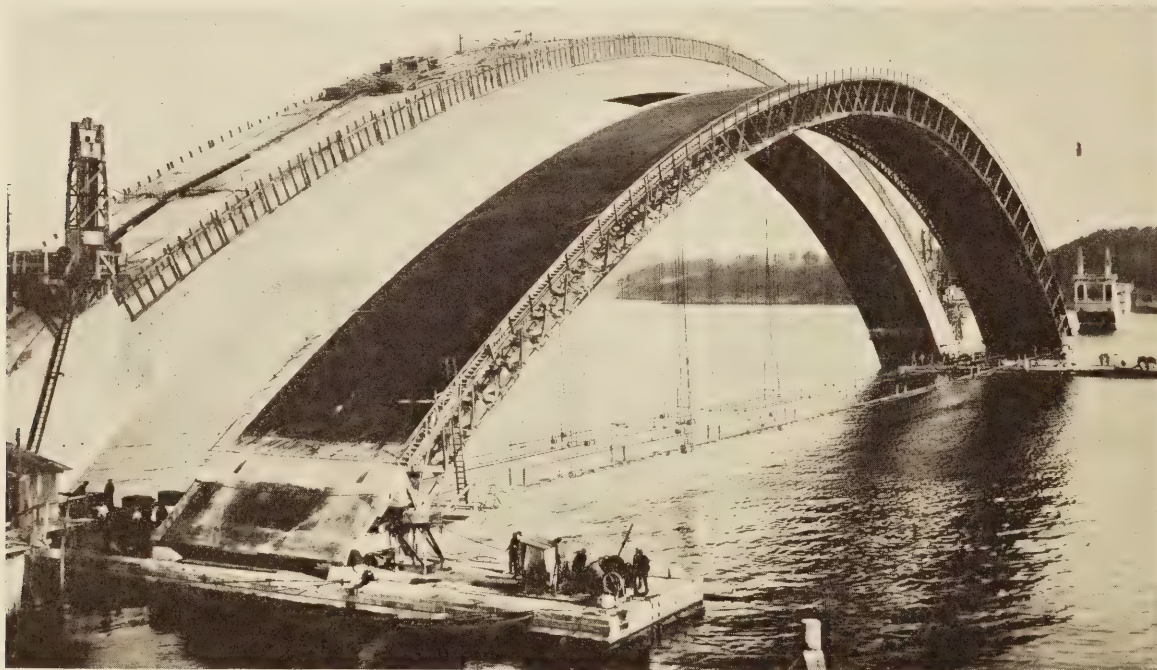
AN ARCH CONSTRUCTED BY THE FREYSSINET METHOD
