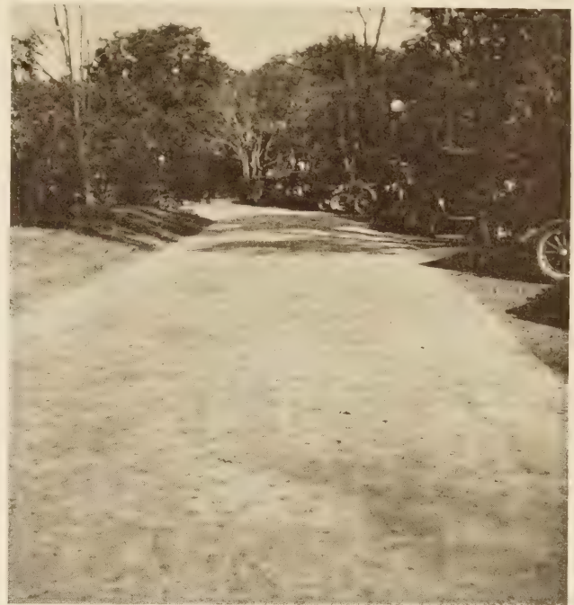
FIGURE 8.—LOCATION AND PRESENT CONDITION OF SECTION 4. THE SURFACE MAT, ALTHOUGH INTACT, IS VERY LIFELESS IN APPEARANCE, DUE TO INSUFFICIENT TRAFFIC
