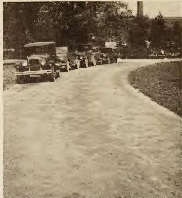
FIGURE 4.—PRESENT APPEARANCE OF SECTION 1. PARKING OF CARS ON ONE SIDE LEAVES ONLY A SINGLE TRAFFIC LANE FOR THE ONE-WAY TRAFFIC
