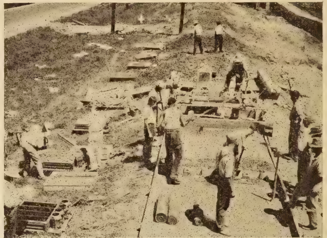
PLACING CONCRETE SLABS AND CASTING SPECIMENS
