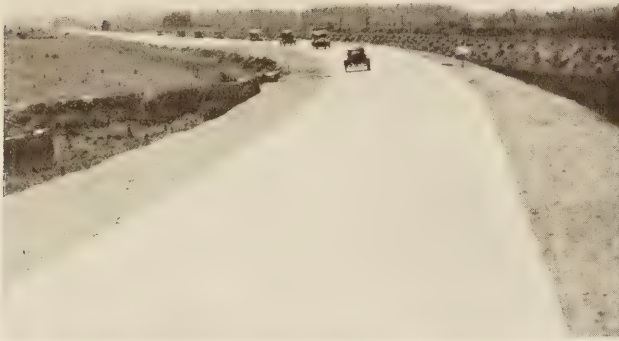
FIGURE 26.—CONCRETE ROAD 20 FEET WIDE DIVIDED BY MEANS OF GROOVES AND JOINTS INTO SECTIONS 10 FEET BY 20 FEET
