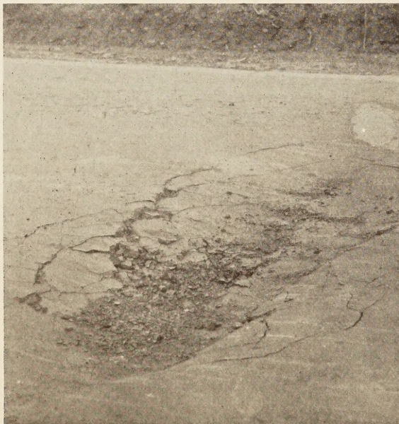
FIGURE 5.—RESULT OF FAILURE OF CONCRETE BASE (LEFT) AND MACADAM BASE (RIGHT). IN BOTH CASES THE SURFACE IS OF THE FLEXIBLE TYPE
