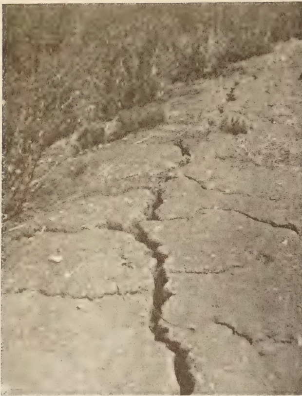
FIGURE 18.—SHRINKAGE CRACKS IN HEAVY CLAY SOIL
