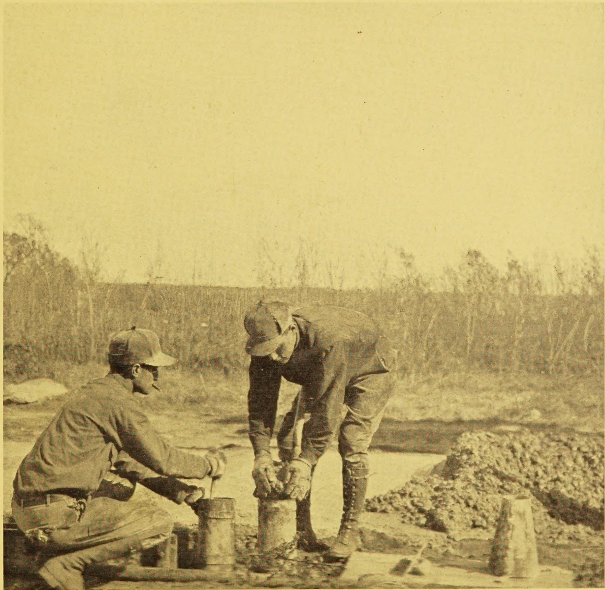
MAKING CYLINDERS AND SLUMP TEST IN STUDIES OF MIXING TIME
