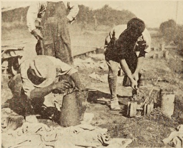
MAKING SLUMP TEST AND CASTING BEAMS ON OKLAHOMA FEDERAL-AID PROJECT 148E
