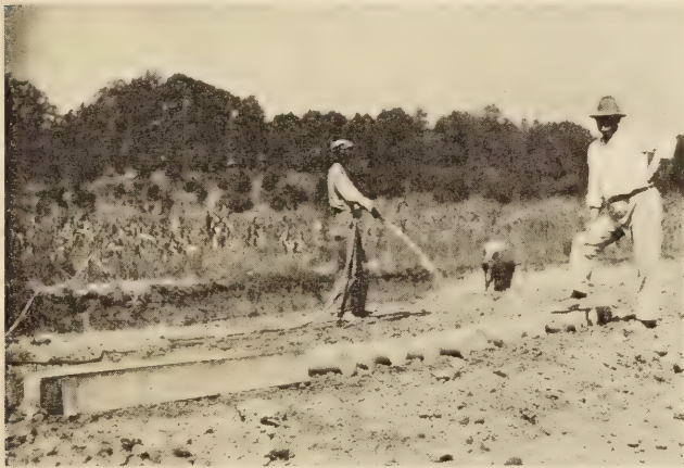
A DAY'S RUN OF BEAMS AND CYLINDERS, ANDERSON COUNTY, TENN.
