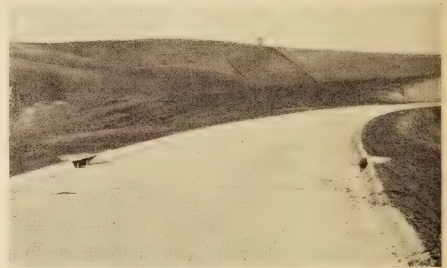
TYPE OF CURB USED BY IOWA IN 1925. NOTE BERM SLOPING TOWARD PAVEMENT
