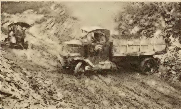
ROAD CONDITIONS HAVE AN IMPORTANT BEARING ON THE EFFICIENCY OF TRUCK HAULING, PARTICULARLY WITH THE LARGER SIZES OF TRUCKS
