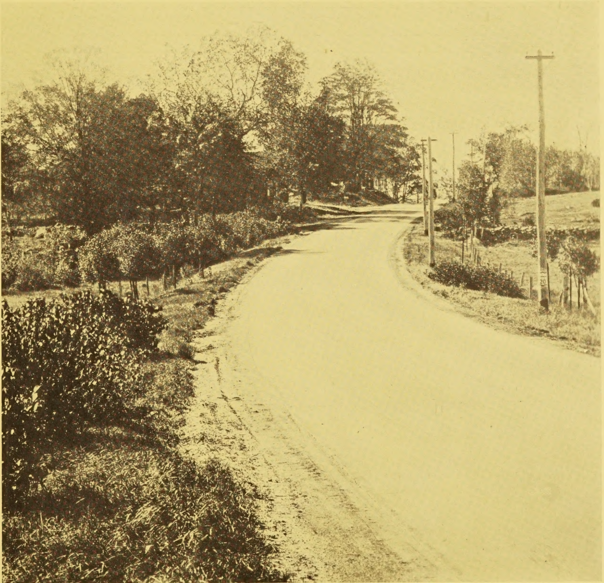
ROADSIDE TREATMENT ON A MASSACHUSETTS STATE HIGHWAY
