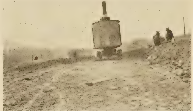
SMOOTH ROADWAY SURFACE LEFT BY A CAREFUL SHOVEL OPERATOR
