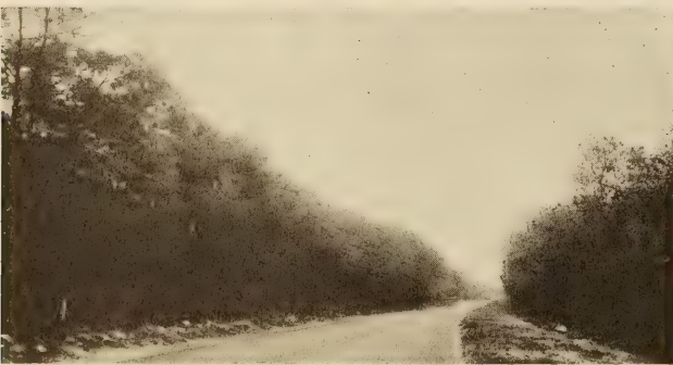
AN EXAMPLE OF WHAT CAN BE DONE BY REMOVAL OF TELEPHONE POLES AND WIRES. THE WIRES SHOWN IN THE UPPER PICTURE ARE CARRIED IN A CABLE SHOWN AT THE LEFT IN THE LOWER PICTURE
