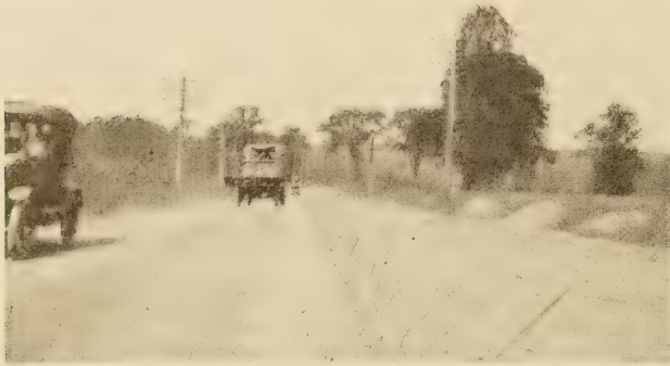
HALF-WIDTH CONSTRUCTION OF CONCRETE PAVEMENTS AVOIDS DETOURING DURING CONSTRUCTION
