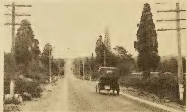
OLD PENETRATION MACADAM IN MARYLAND RECONSTRUCTED AND WIDENED BY THE ADDITION OF NEW CONCRETE SHOULDERS AND NEW PENETRATION MACADAM TOP
