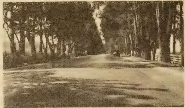
A CALIFORNIA ROAD, ORIGINALLY A 24-FOOT BITUMINOUS CONCRETE ON A CONCRETE BASE, WIDENED TO 42 FEET BY THE ADDITION OF CONCRETE SHOULDERS AND A NEW ASPHALTIC CONCRETE SURFACE APPLIED
