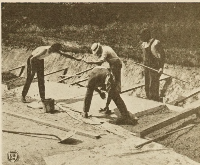
Finishing the concrete
