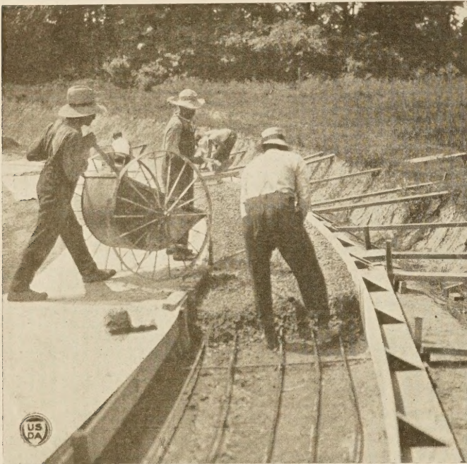
Placing the concrete
