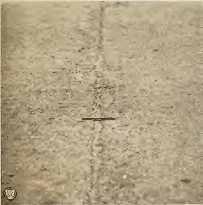
The light-colored material fills the joints well, does not bleed, and has outlasted two fillings with asphalt
