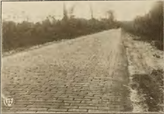
FIG. 4.—Bituminous-filled relaid brick surface between Jacksonville and Atlantic Beach, giving good service though in the first stage of deterioration.
