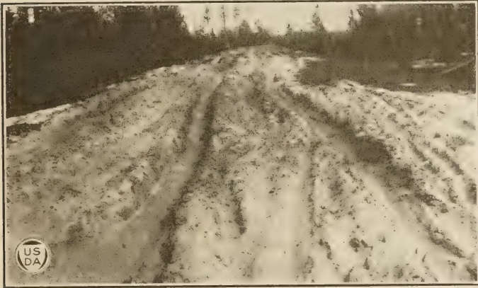
FIG. 1.—Graded natural Florida soil road. State Route No. 2, south of Crescent City.
