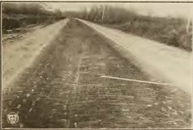
FIG. 11.—Grooves in a narrow sand-filled brick surface between St. Augustine and Hastings.
