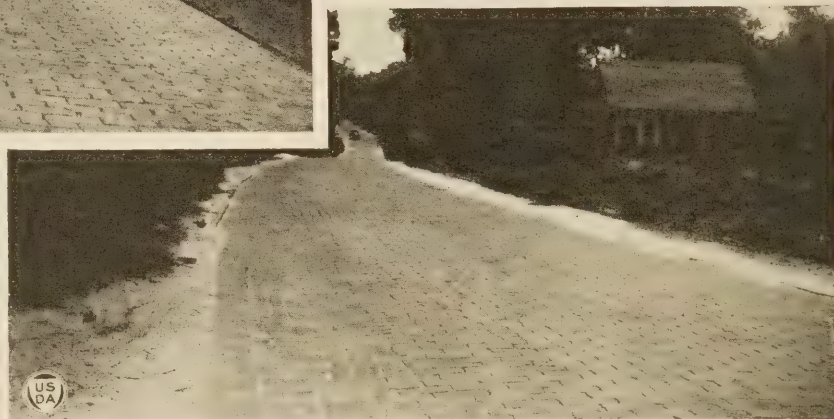
Fig. 10.—(UPPER) SAND-FILLED SURFACE ON STATE ROUTE NO. 4, JACKSONVILLE TO ST. AUGUSTINE, SHOWING DEPRESSION OF THE EDGES OF THE PAVEMENT. (LOWER) ANOTHER VIEW OF THE SAME ROAD SHOWING MARKED UNEVENNESS.
