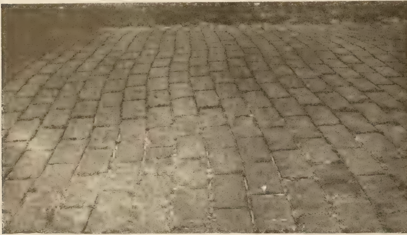
FIG. 13.—(UPPER) LONGITUDINAL MOVEMENT OF BRICK IN THE ORANGE PARK ROAD. NOTE GRASS GROWING IN THE SAND FILLER. (LOWER) TRANSVERSE SEPARATION OF BRICK PERMITTED BY SPREADING OF CURBS.
