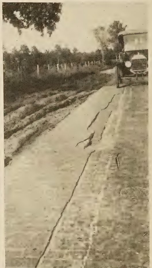
FIG. 19 (RIGHT).—THIS BREAK COULD NOT HAVE OCCURRED HAD NOT THE SAND SUBGRADE BEEN DISPLACED.
