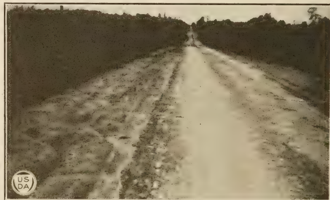
FIG. 27.—Limerock road compacted by road roller. Built in 1913 and carefully maintained, it is now a very satisfactory, hard, and compact road.
