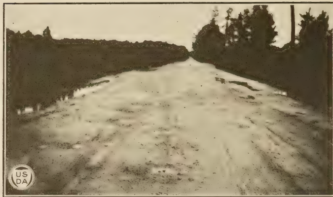
FIG. 26.—Limerock road compacted by traffic. Laid in 1914.
