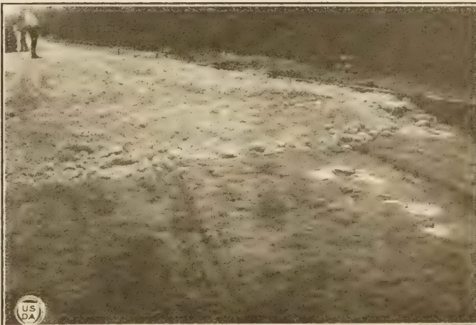
Fig. 24.—Limerock base before rolling.
