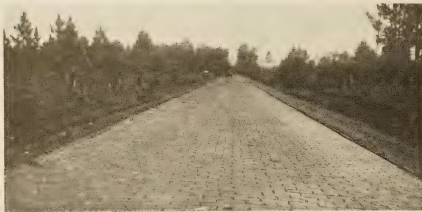
Fig. 10.—(UPPER) SAND-FILLED SURFACE ON STATE ROUTE NO. 4, JACKSONVILLE TO ST. AUGUSTINE, SHOWING DEPRESSION OF THE EDGES OF THE PAVEMENT. (LOWER) ANOTHER VIEW OF THE SAME ROAD SHOWING MARKED UNEVENNESS.
