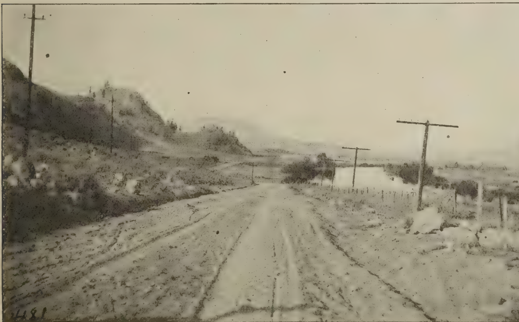
WASHINGTON FEDERAL-AID PROJECT NO. 14, IN OKANOGAN COUNTY, SURFACED WITH SCREENED GRAVEL
