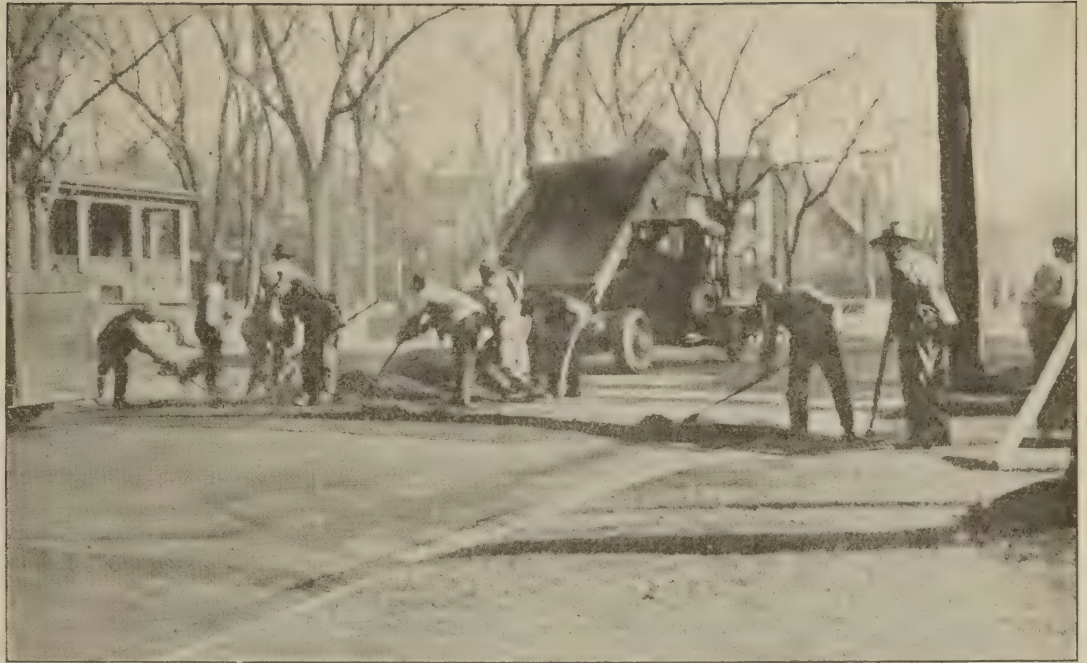
LAYING THE SHEET ASPHALT TOPPING.
