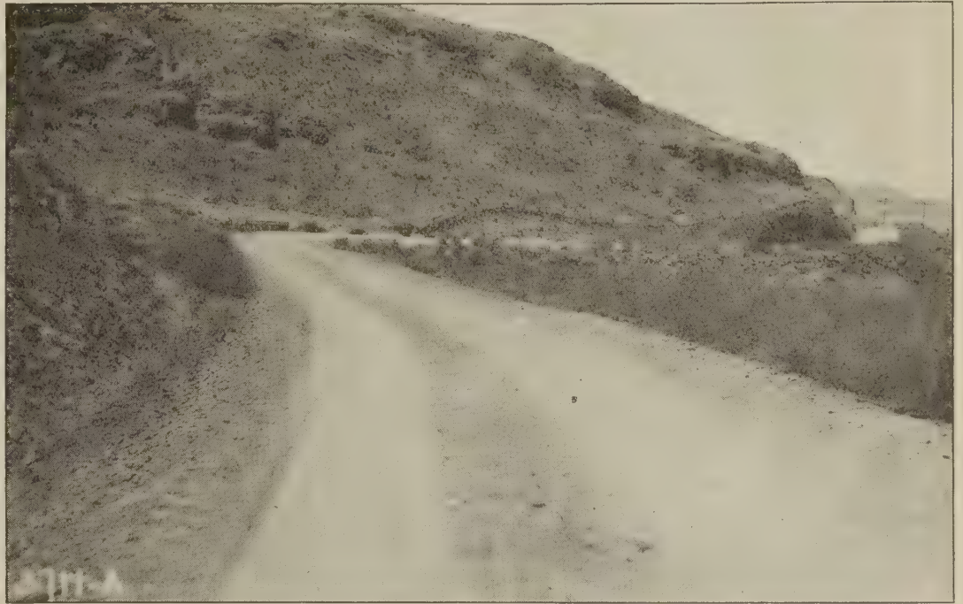
FEDERAL-AID PROJECT NO. 44, IN GILLIAM COUNTY, OREG., SURFACED WITH CRUSHED GRAVEL
