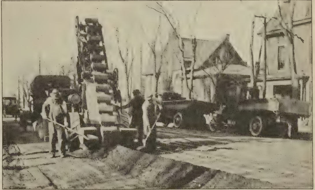
REMOVING THE EXCESS MATERIAL AFTER SCARIFYING THE OLD MACADAM.
