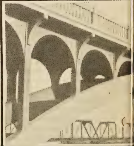
CONCRETE BRIDGE NEAR
