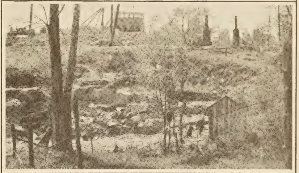
TOP: ECONOMICAL ARRANGEMENT OF CRUSHER PLANT. STONE RUNS TO CRUSHER BY GRAVITY. BOTTOM: EXPENSIVE WAY OF GETTING ROCK TO CRUSHER.
