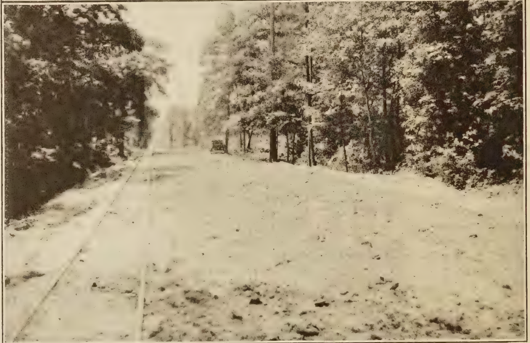
TOP—SHOWING CONCRETE WITH A STEEL TEMPLATE. BELOW—SHOWING EARTH BLANKET WHICH IS KEPT ON FOR THIRTY DAYS.
