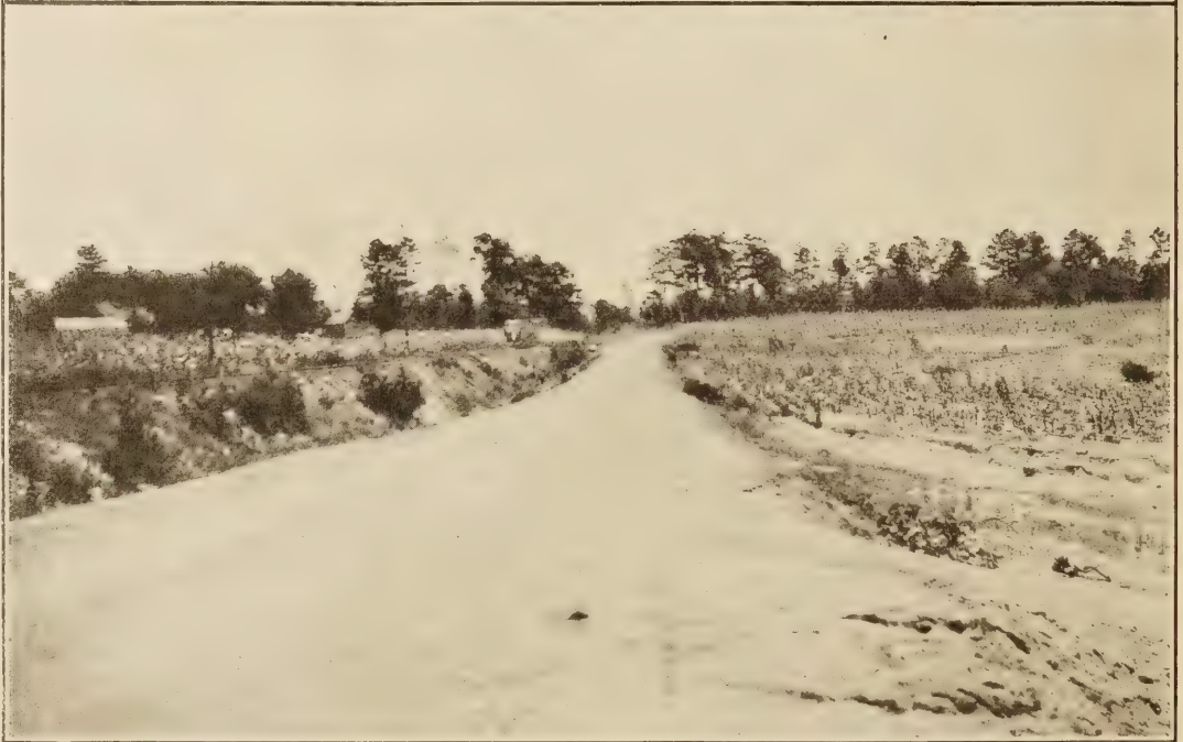
THE OLD AND THE NEW. AT THE TOP TAKEN OPPOSITE THE POINT ILLUSTRATED BELOW IS SHOWN A LOOSE SAND ROAD IN DALE COUNTY, ALA., THE SAND BEING 10 INCHES DEEP AND THE ROAD LITTLE MORE THAN A CHANNEL FOR DRAINAGE. BELOW—THE NEW NATURE-MIXED SAND-CLAY HIGHWAY.
