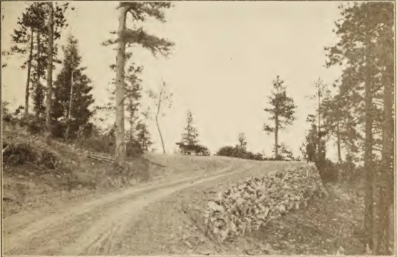
SWITCHBACK ON SECTION OF SEDALIA-DECKER SPRINGS ROAD, PIKE NATIONAL FOREST, COLORADO.
