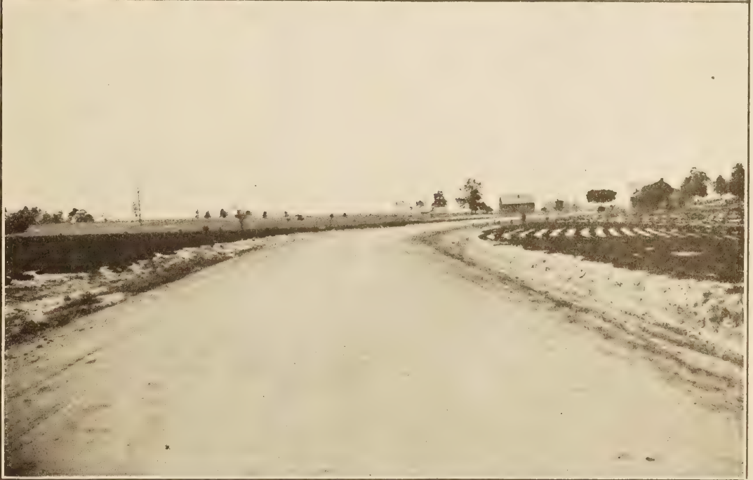
ALABAMA'S FIRST COMPLETED FEDERAL AID PROJECT. NATURE-MIXED SAND-CLAY ROAD IN PIKE COUNTY. THE PEANUT CROP OF THIS COUNTY IN 1917 WAS WORTH $2,000,000.
