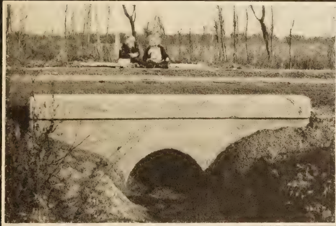
TOP, LEFT—BRIDGE AND CATTLE PASS, CALHOUN COUNTY, ALA., COST $250. TOP, RIGHT—STONE CULVERT IN CHICKAMAUGA PARK, TENNESSEE. BOTTOM, LEFT—HALF ARCH CULVERT IN POTTAWATOMIE COUNTY, OKLA. BOTTOM, RIGHT—CULVERT WITH FLAT STONE TOP AT BRUNSWICK, MAINE.
