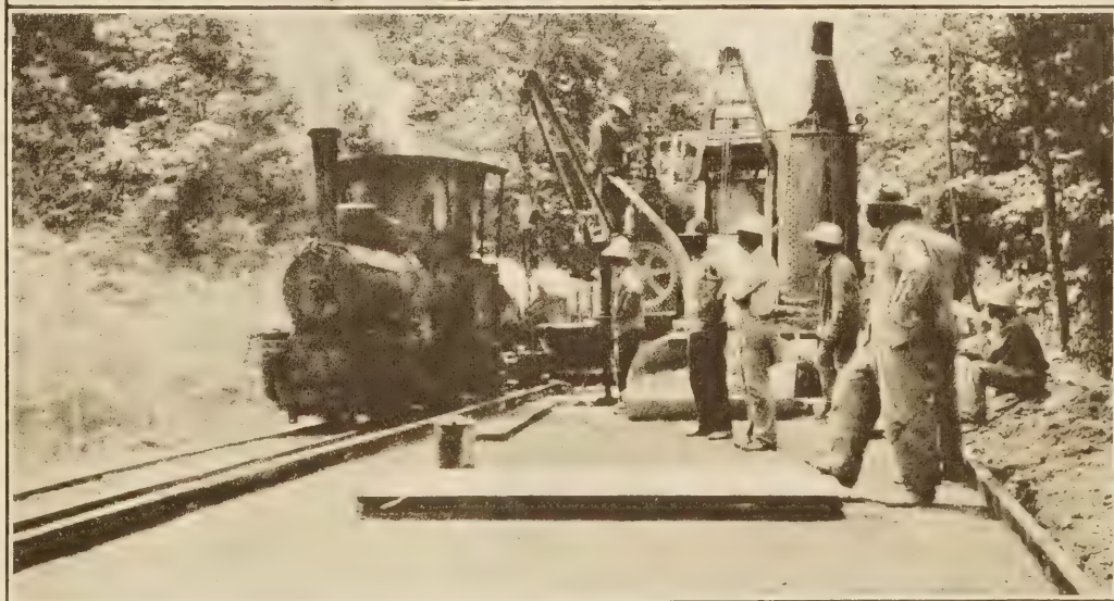
THE OLD METHOD AND THE NEW. DUMPING MATERIAL ON THE GRADE AND HANDLING BY DIRECT LOADING WITHOUT LOSS AND AT A SAVING IN TIME AND LABOR.
