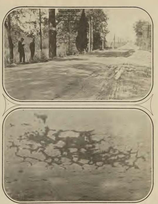
TOP - WATER STANDING IN MUD HOLE ON SHOULDER AT EDGE OF PAVEMENT ON 5-FOOT FILL, BOTTOM - MOISTURE BEING SHOVED THROUGH FROM BASE OPPOSITE MUD HOLE SHOWN AT TOP.
