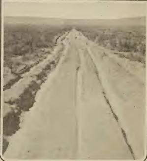
AT TOP-NATURAL SOIL ROAD IN NEVADA, WHICH BECAUSE OF THE EXCELLENT GRAVELLY SOIL IN WHICH IT IS LOCATED REQUIRES BUT LITTLE MAINTENANCE AT BOTTOM-ROAD ACROSS LOW ALKALI FLAT WHICH BECAUSE OF THE SILTY SOIL IN WHICH IT IS LOCATED AND THE LONG DRY SUMMER RAPIDLY GUTS UP UNDER TRAFFIC. THIS ROAD HAS BEEN RELOCATED IN BETTER MATERIAL.
