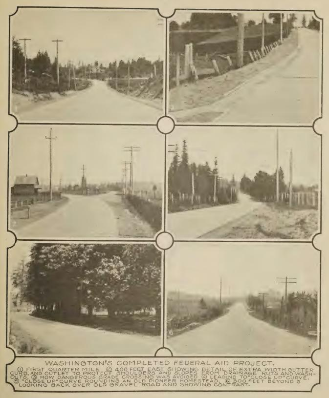
shoulders, nowhere less than 5 feet wide. Altogether the project includes a broad-guage pavement on an ample roadbed. The grade maximum is 5 per cent, the general project being level, with undulations varying not to exceed 50 feet in their extremes.
