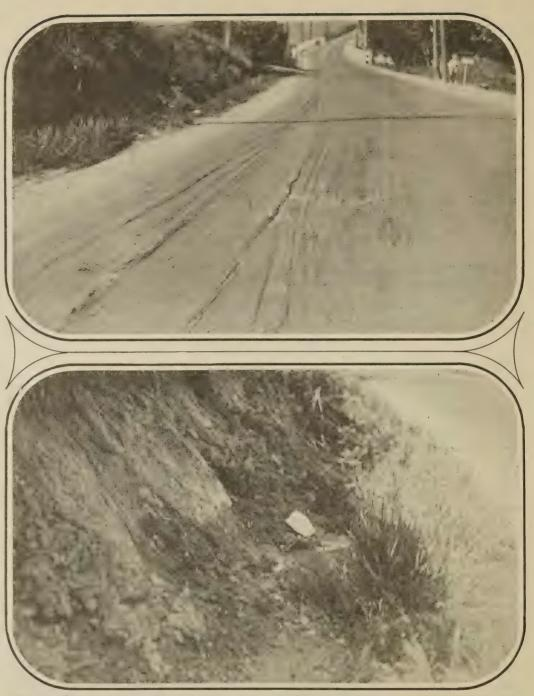
TOP-FAILURE IN 6-INCH CONCRETE ROAD DUE TO SOFTENING OF SUBGRADE BY WATER BEING AB-SORBED FROM DITCH WHICH HAS BEEN FILLED UP AND NOT CLEANED DUT. BOTTOM- WATER STANDING IN DITCH OPPOSITE FAILURE SHOWN ABOVE.
