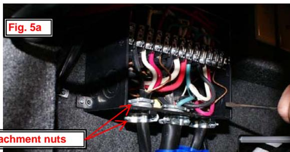
6. Loosen wire attachment set screws and disconnect all 3 power cords from the transfer switch terminal strip. Disconnect and remove the bare copper bonding ground wire.
