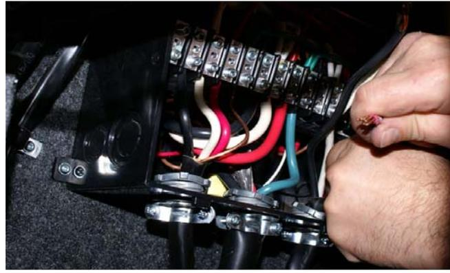
8. Remove the existing transfer switch from the compartment wall. Retain the mounting screws for re-use.
