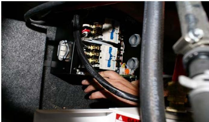
12. Connect the single bare copper bonding ground wire (from the chassis frame) to the bottom left buss bar on the transfer switch box. NOTE: This bonding wire enters the box through a small hole which aligns with a specific buss bar cavity.
