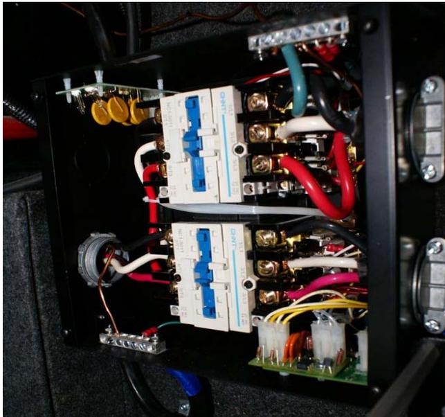
17. Tighten the Romex saddle clamps to provide cable strain relief. Do not overtighten.
