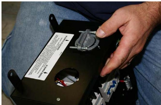
11. Using the original (4) screws, install the new transfer switch so that the shore line and generator inputs point toward the outside wall of the motorhome. NOTE: The original switch was mounted with wire entry from the bottom side. The new transfer switch must be installed so that wire entry is from the sides of the box. Power cables may need to be relocated to make room for the new switch.
