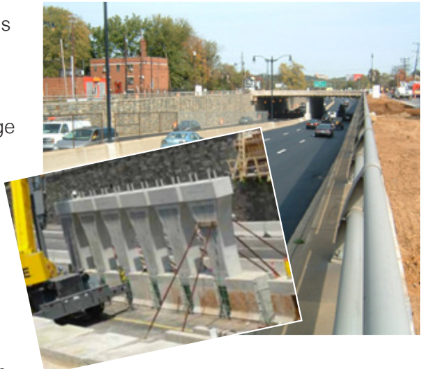
The new, taller bridge is expected to reduce clearance-related crashes and be safer for drivers and pedestrians. (Inset) Using prefabricated pier units helped the District DOT finish the project faster.
