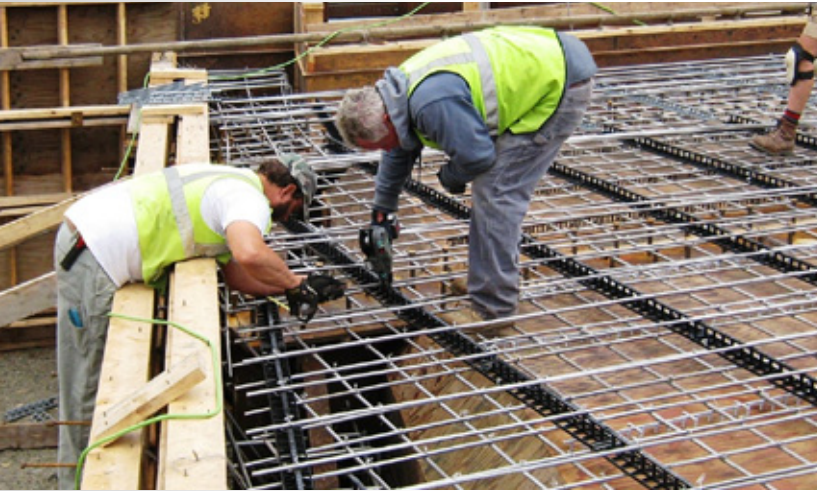
Crews used stainless steel rebar to reinforce a bridge superstructure on a Highways for LIFE project in Vermont.
