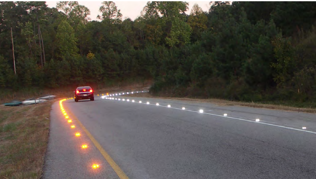
LED raised pavement markers, a safety technology undergoing a Technology Partnerships study, are designed to increase the visibility of roadway curves so drivers can navigate them more easily.
