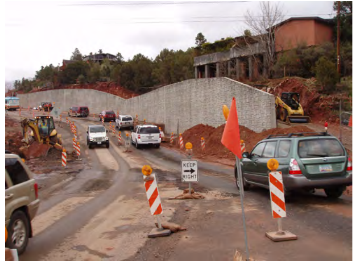
States are using innovative construction techniques and contracting methods to improve work zone mobility and safety.
